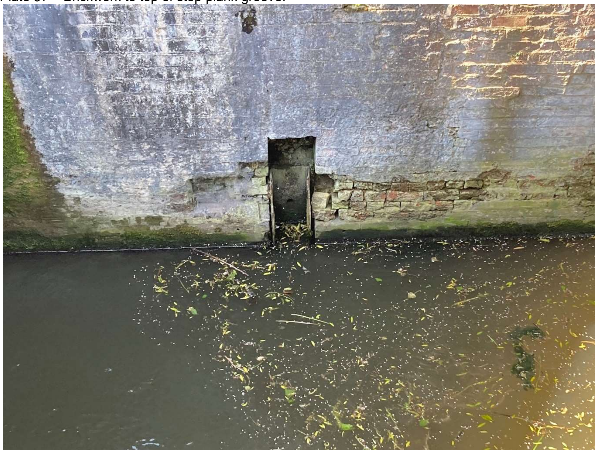
Plate 57 – Brickwork to top of stop plank groove.
