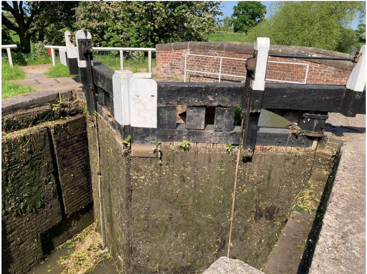
Plate 56 – Bottom end lock gates upstream face
