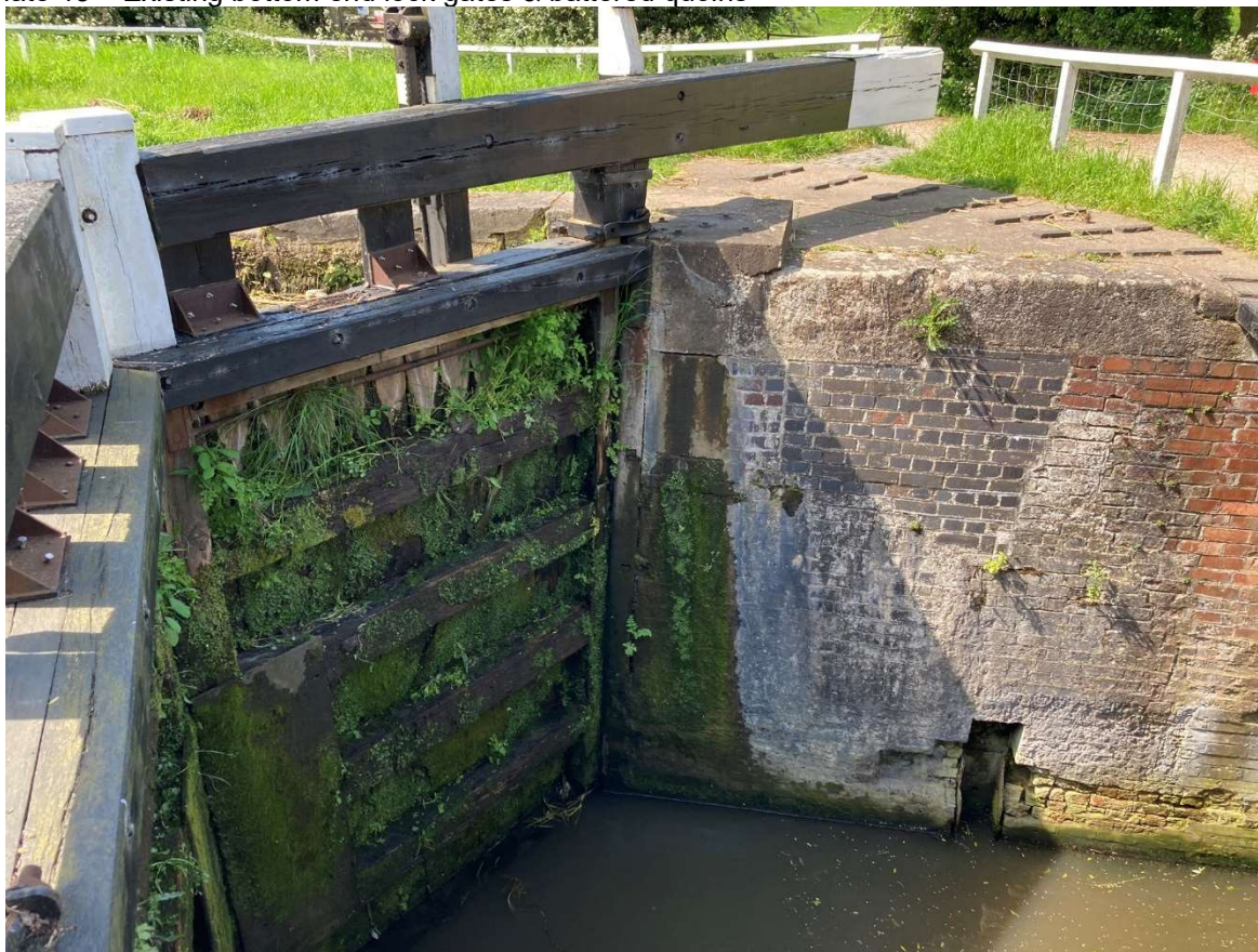
Plate 46 – Existing bottom end lock gate balance beams & footbridge
