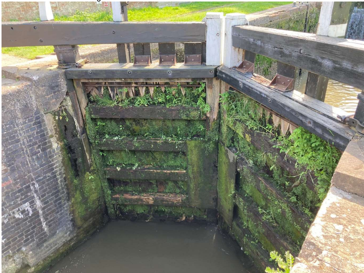
Plate 55 –Bottom end lock gates downstream face
