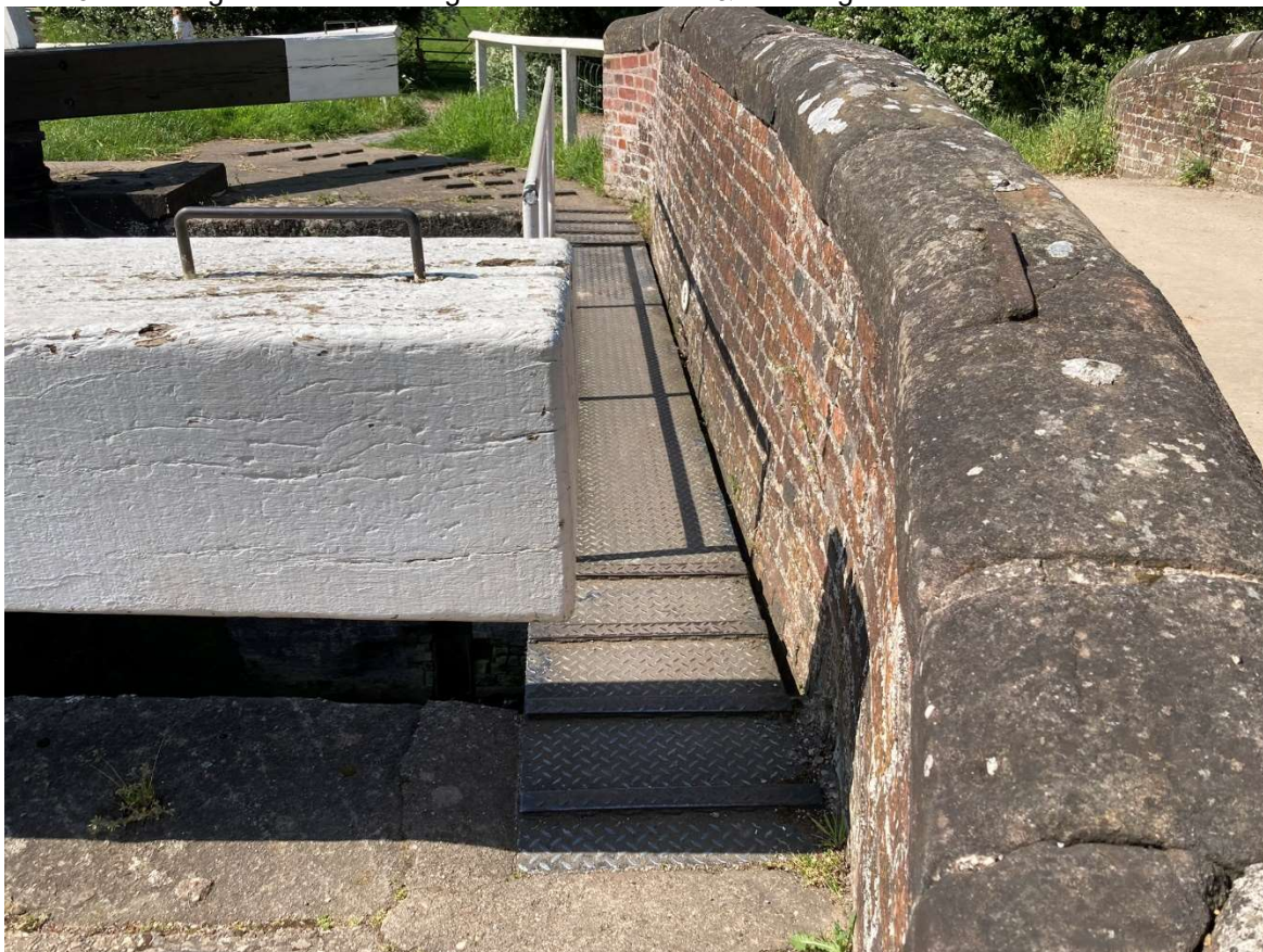
Plate 46 – Existing bottom end lock gate balance beams & footbridge
