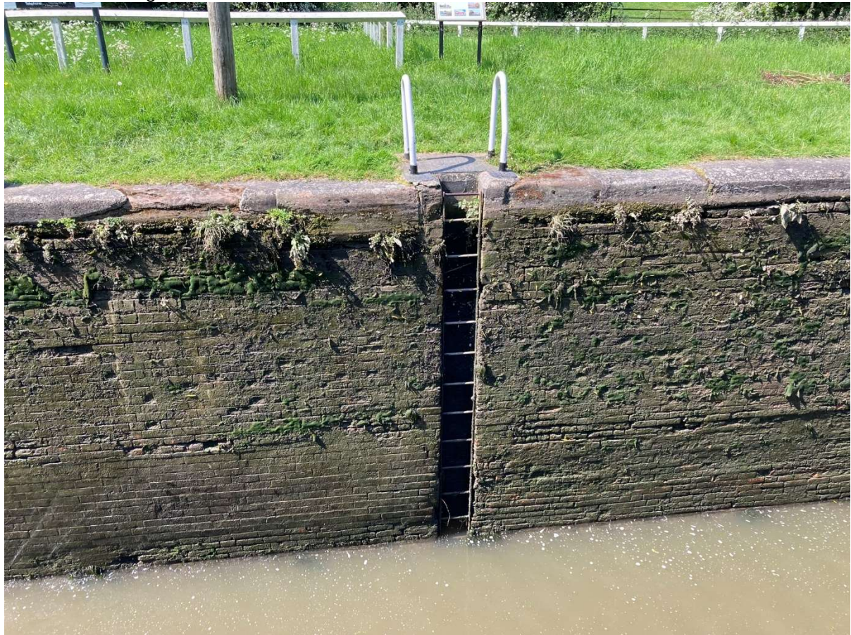
Plate 49 – existing offside lock ladder
