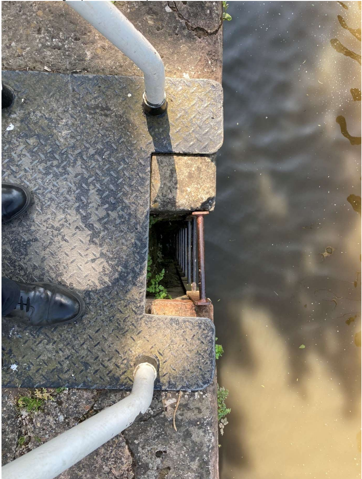
Plate 48 – existing towpath lock ladder top
