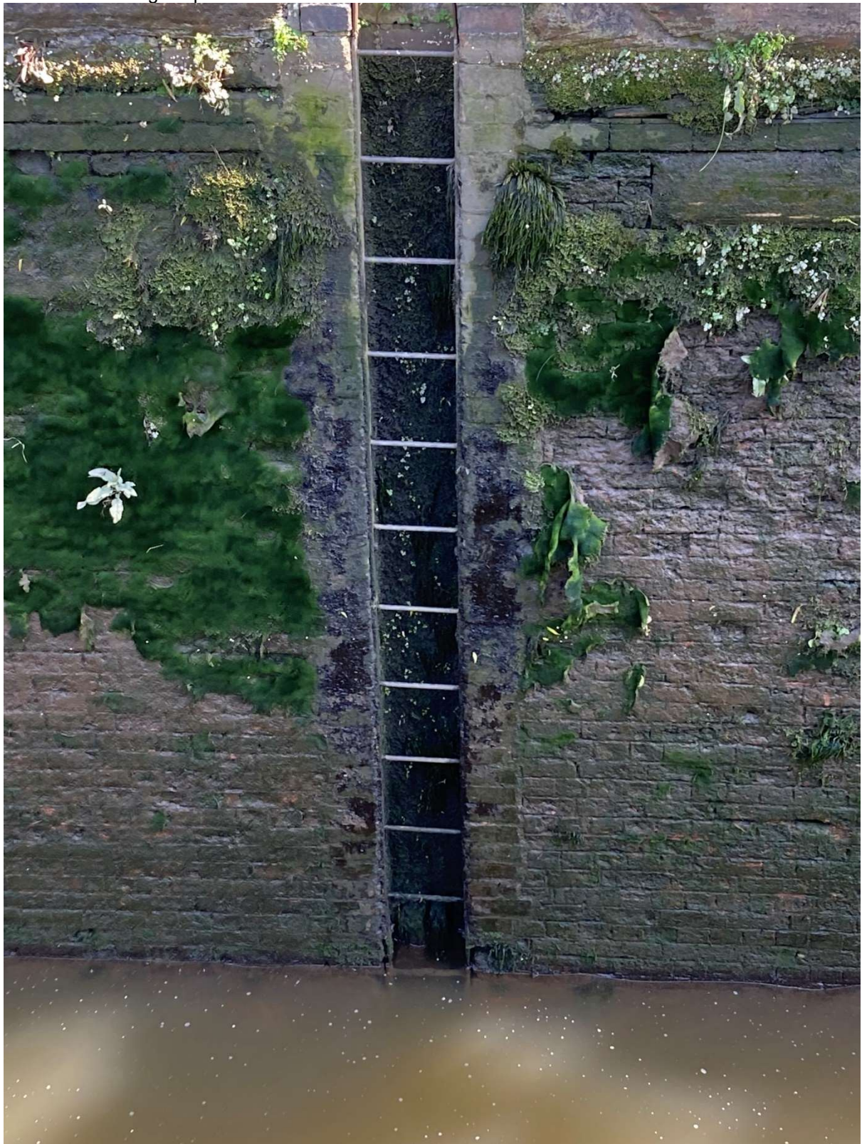
Plate 47 – existing towpath lock ladder
