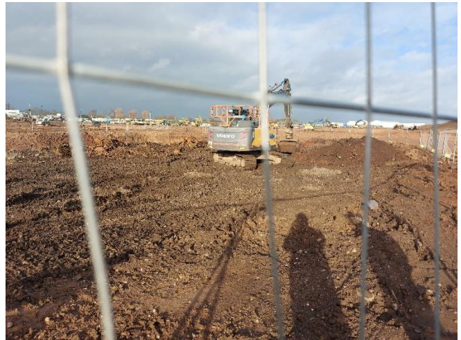
U9 towards North – Marl Pit excavation has resumed.
