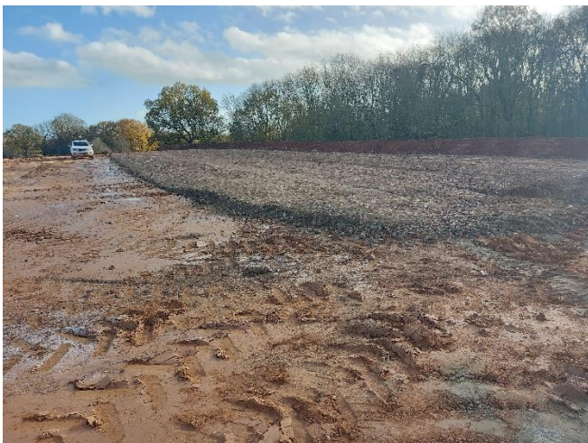
AA7 towards East – Working platform completed for crane operations to install Retaining Wall RW3.
