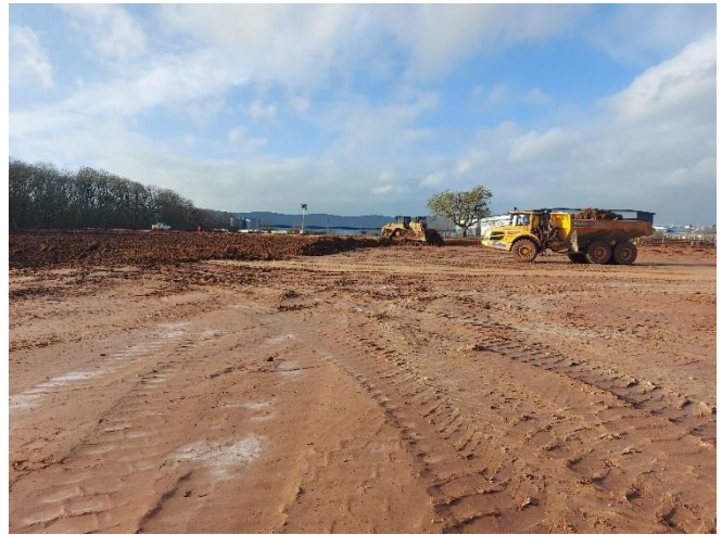
X12 towards West – Fill placement is ongoing at grids X10-X11 and Y10-Y11.
