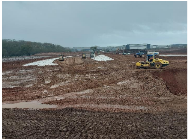
T16 towards west - Lime stabilisation underway in fill areas at grids W11–W15, X11–X13, and V11–V14.
