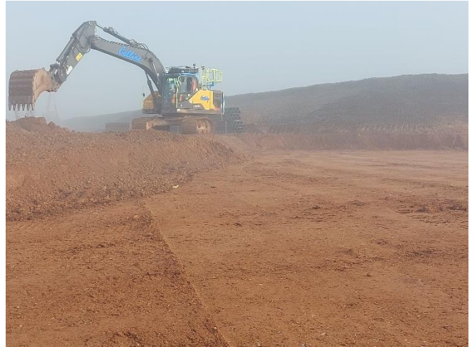
N8 towards east - Excavation for roundabout at grids N9-N10 is ongoing.
