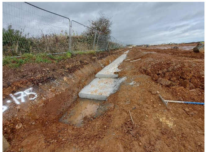
V3 towards North – Retaining Wall RW3 foundation has been completed.
