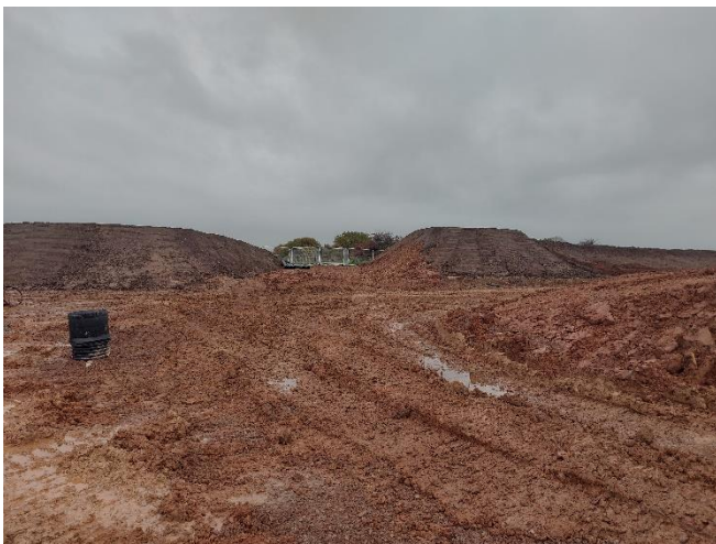
H9 towards East (H10) – Landscape bund is partly removed to install the drainage – to be reinstated.
