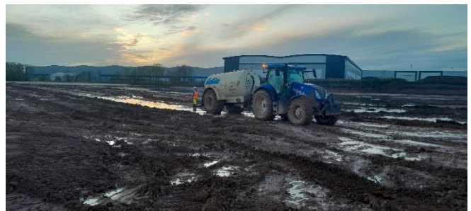
Grid R6 towards East-southeast – Pumping of surface water.
