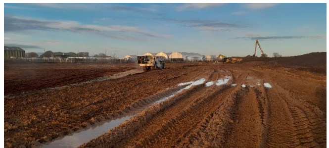
Looking toward Grids J-L;7&8 (North-northwest) – Rotovating/mixing.
