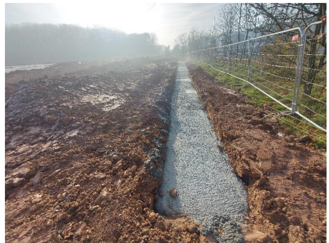
Z3 towards south – Retaining Wall RW2, foundation casting has been completed.
