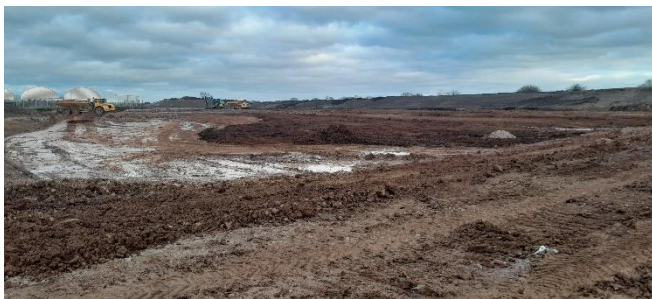
Looking toward Grids J-L;6-8 (North-northeast) – Borrow pit.
