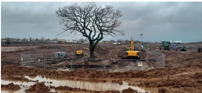
Grid Y;9 towards North – Tree removal is still ongoing.
