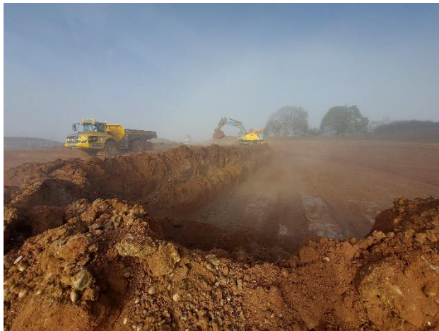
U15 towards north - Pond excavation continues at grids S14-S15 and T14-T15.
