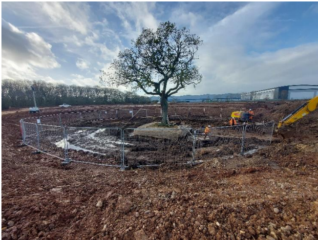
X10 towards West – Tree removal is still ongoing.
