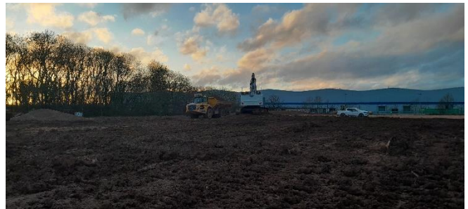
Looking toward Grids Z;8 (Southwest) – Overfill being trimmed, and supplying retaining wall backfill.
