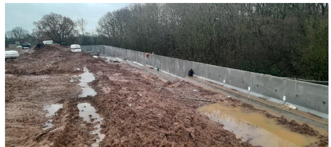
Grid AA;6 towards East-southeast – Installed retaining wall stems.
