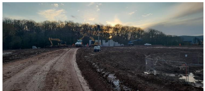
Looking toward Grids AA;7&8 (south-southwest) – Mobilisation to site of retaining wall materials.
