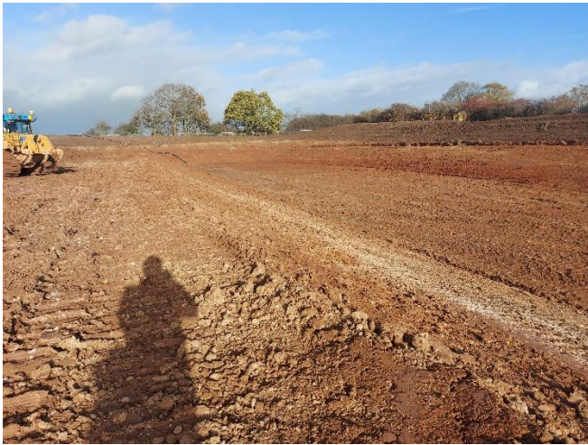
U14 towards Northeast – Pond excavation has been completed.
