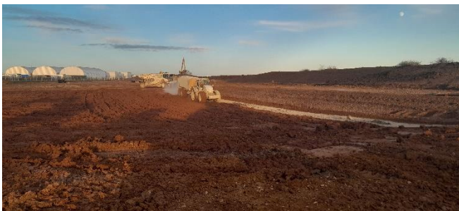
Looking toward Grids J-L;7&8 (North-northeast) – Lime spreading.
