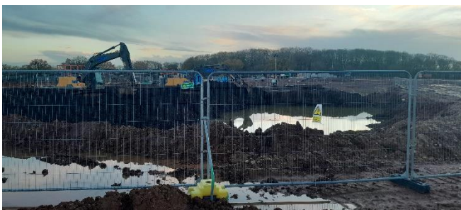
Grid Q6 towards Southeast – Resumed pond excavation.
