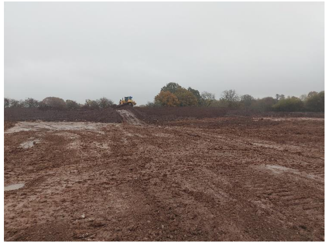
Landscape bund construction is currently underway at grids V17/W18 following a 2-week hold period.
