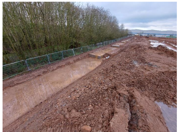
AB10 towards west – Completed foundation section of Retaining Wall 3.
