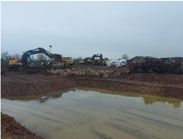
N5 towards northwest – Screening of large objects from material excavated from deeper area of Marl Pit is ongoing.
