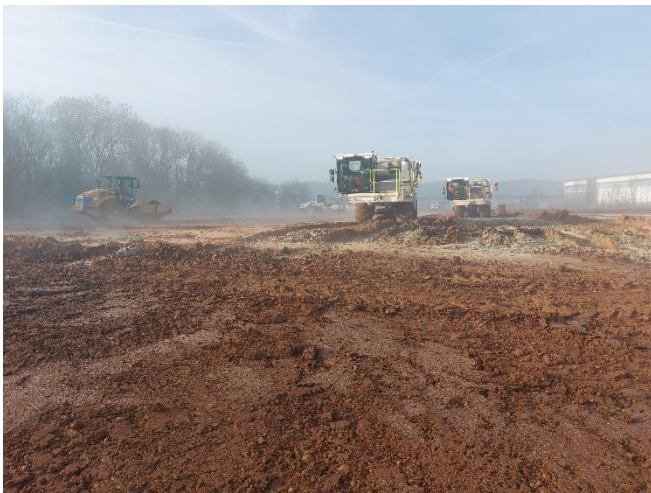
Z10 towards northwest - Cement stabilization is ongoing at grids Z7-Z10 and AA7-AA10
