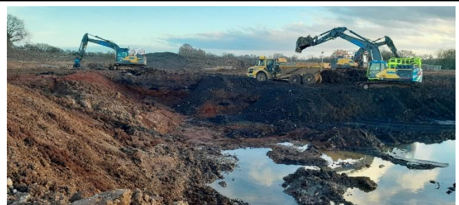
Grid S;6 towards Southeast – Pond excavation.
