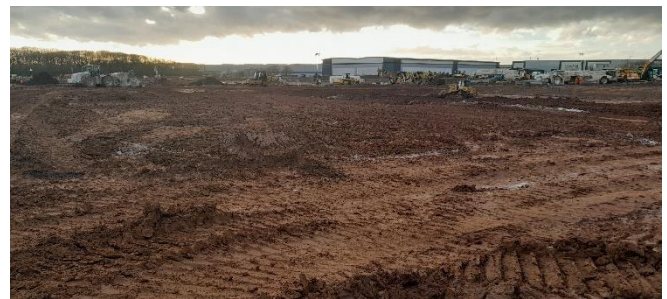
Looking toward Grids J-L;6-8 (South-southwest) – Borrow pit.
