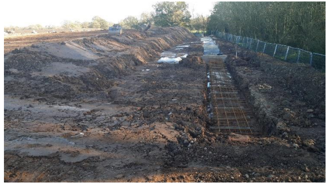
AB7 towards east - Retaining Wall 3 foundation partially cast; remaining sections at grids AB7-AB8 and AA10 scheduled for casting today.
