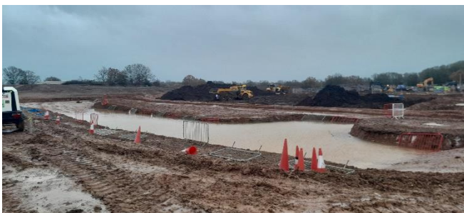
Grid M;6 towards South-southeast – Surface water conditions.
