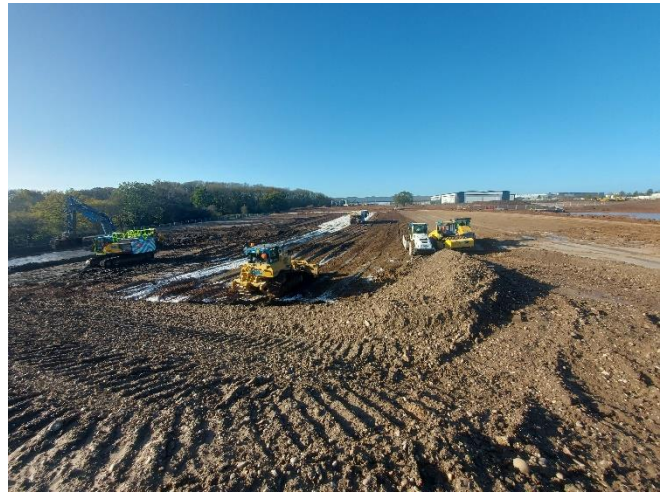
U17 towards West - Lime stabilisation underway in fill areas at grids V11–V14, W11–W15 and X11–X13.
