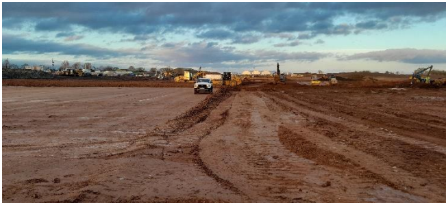
Grid U;6 towards North – Trimmed rerolled/treated ground (Grids W-AA;4-6)
