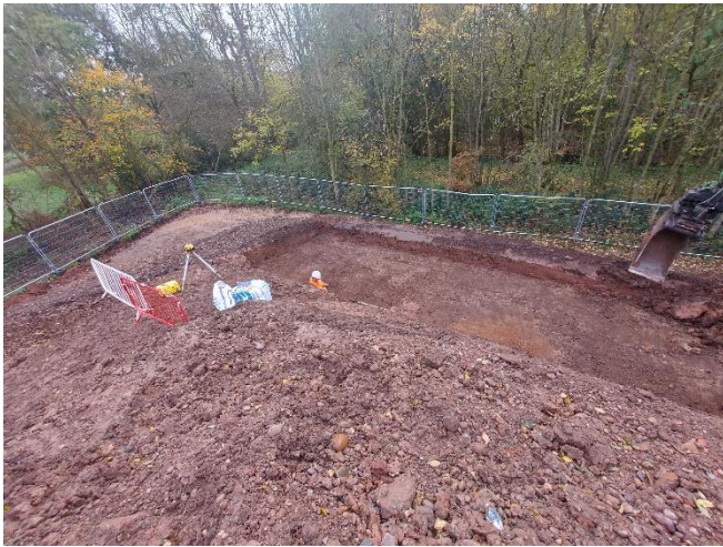
AB9/AB10 - Formation of retaining wall foundation currently being prepared.
