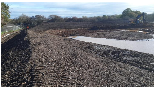
R13 towards S14/S15 – Pond excavation in progress at grids S14–S15.
