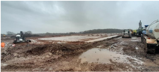
Grid N;3 towards South-southeast – Overview.
