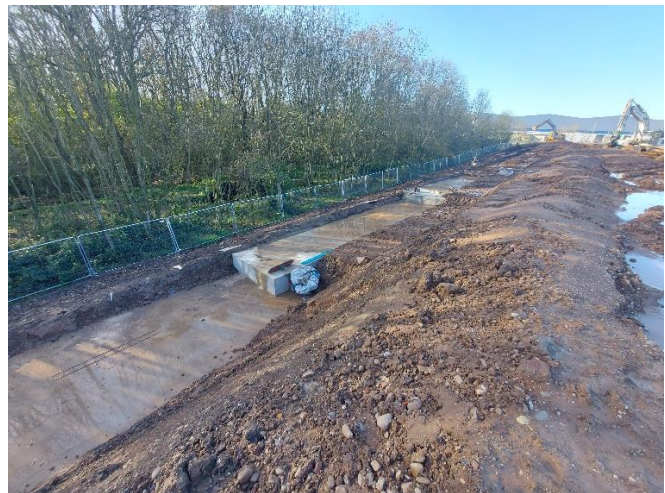
AB7 towards east - Retaining Wall 3 foundation partially cast at grids AB9-AB10.
