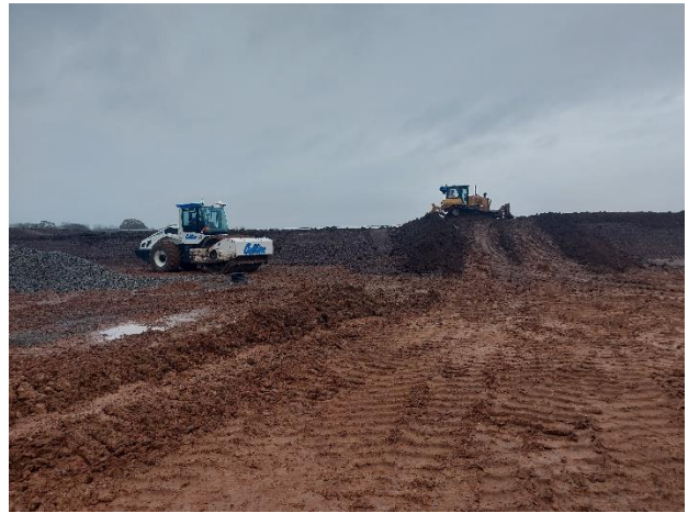
F8 towards east - Landscape locally excavated for drainage works at grids F10/G10 currently being reinstated, almost nearing completion.
