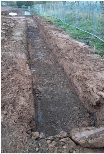
X3 towards south –Retaining Wall 2 foundation approximately 50% cast.
