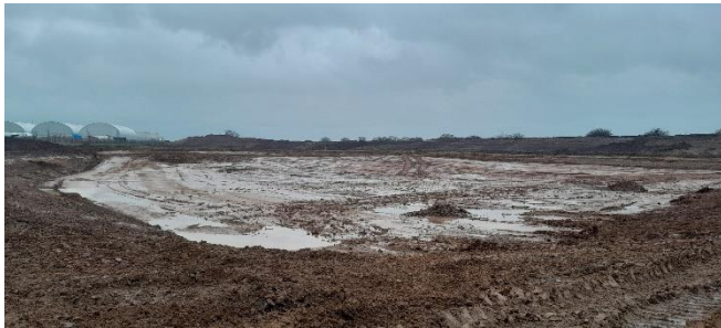
Looking toward Grids K&L;6-8 (North-northeast) – Borrow pit (work paused but infill prior to visit).
