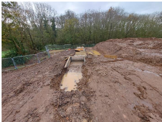
Z10 towards south – Final remaining section of the Retaining Wall 3 foundation yet to be completed in grid Z10 to AA10.
