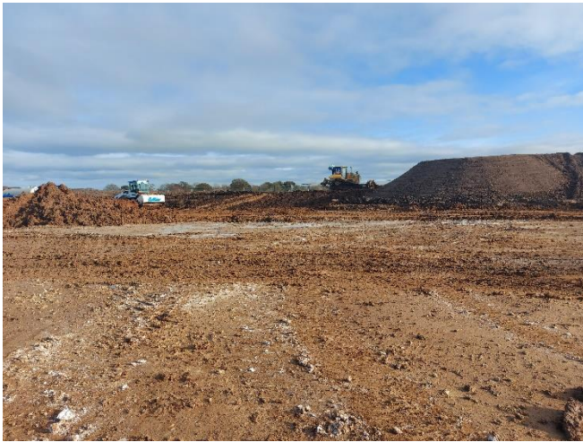
G9 towards East (F10) –Partly removed landscape bund to install the drainage currently being reinstated.
