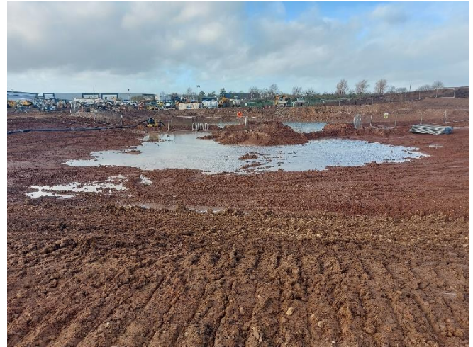
K9 towards West – Water yet to be pumped from the burrow pit to the excavated pond S14-S15 to W16.
