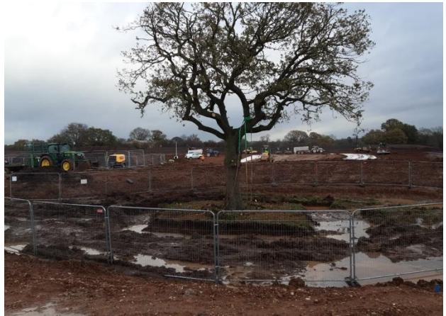
X8 towards east – Preparation works ongoing for tree removal at grid X9.
