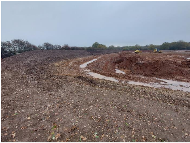
R9 towards southeast – Pond excavation progressed deeper at grids S14-S15.
