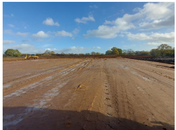
W11 towards East – Fill placement has been completed at grids V12-V14, W12-W14 and X12-X13.
