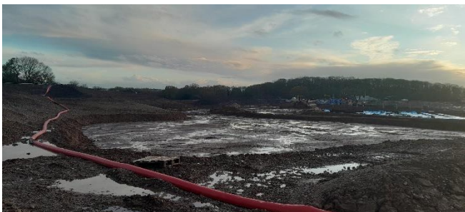
Grid P10 towards South – Pump line from borrow pit to new drainage pond.
