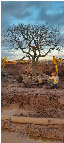
Grid Y;9 towards North – Tree removal is still ongoing.
