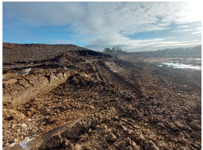
M9 towards east - Landscape bund partially removed at grid M10 to facilitate tree positioning.
