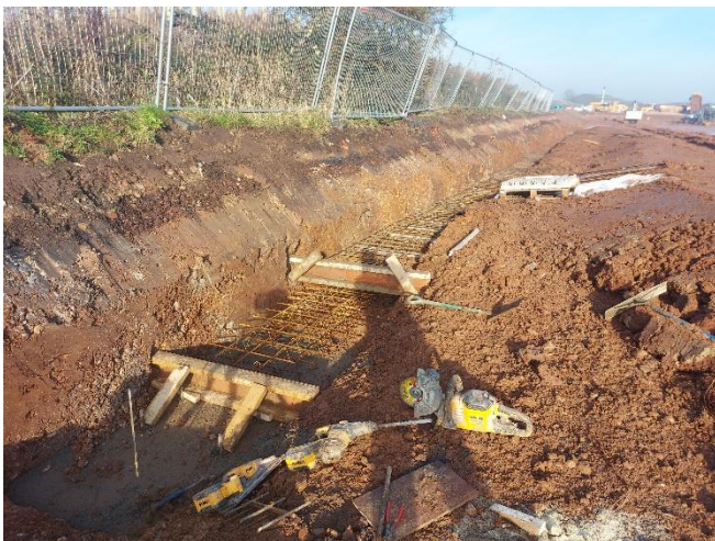
V3 towards north –Retaining Wall 1 foundation yet to be casted – reinforcement is being placed.
