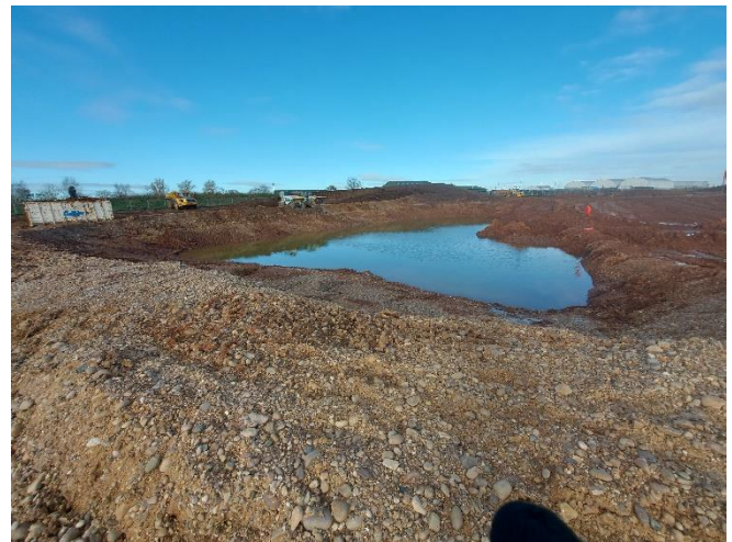
M6 towards North – Infilled Pond / burrow pit in the northern part of site is fully excavated – ponding water is currently being pumped out.
