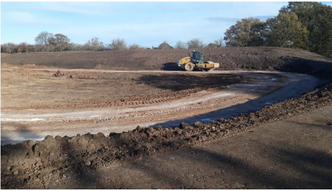
X15 towards east - Fill placement for pond ongoing at grids W15-W17.
