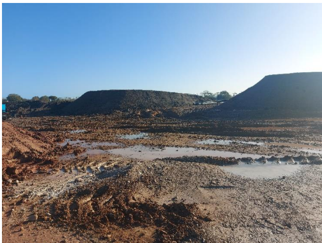
G8 towards East (F10/G10) – Partly removed landscape bund to install the drainage.
