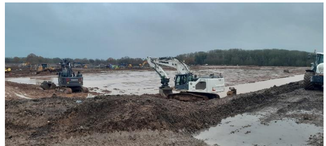
Grid P;4 towards South-southeast – Surface water conditions.
