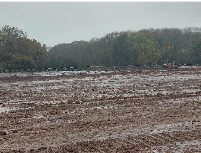
X12 towards Z12/Z13 – Landscape bund construction currently on pause after 4 layers.
