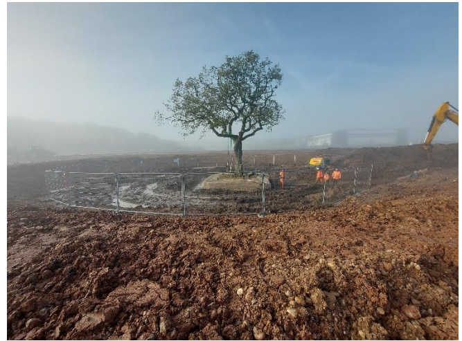
W10 towards west - Oak tree removal works are ongoing at grid W9.
