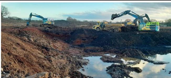
Grid S;6 towards East-southeast – Pond excavation.
