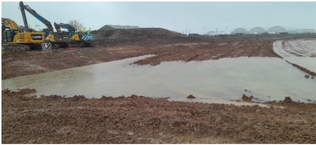
Looking toward Grids J-L;6-8 (North-northeast) – Borrow pit.
