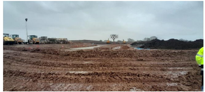
Looking toward Grids M&N;7-11 (Southeast) – Haul/site road and relocated tree.
