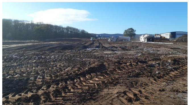
V14 towards West – Lime stabilisation underway in fill areas at grids W11–W15, X11–X13, and V11–V14.
