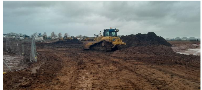
Looking toward Grids Q;8-10 (North-northwest) – New 'Marl Pit' excavation stockpiled.
