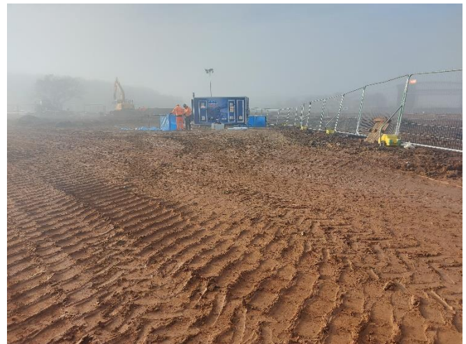
T10 towards east – Decontamination unit is being set up at grid J8-J9 for Marl Pit personnel entry.
