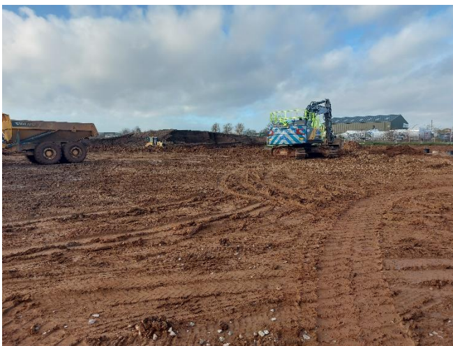
J9 towards North – Reducing level to the north of burrow pit in progress and excavated material being placed as fill at grids X10-X11 and Y10-Y11.
