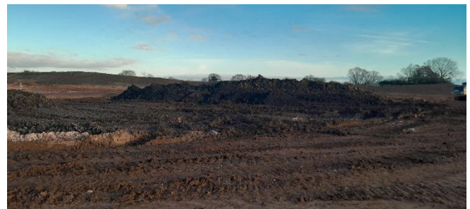
Grids Q;7-10 toward North-northeast – 'Marl Pit' excavation stockpile.
