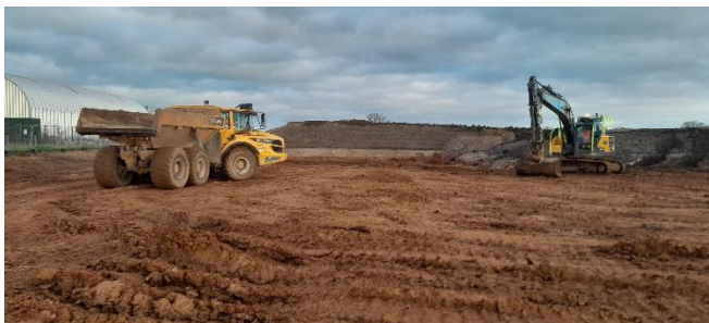
Grid F;9 towards Northeast – Cut and stockpile movement.
