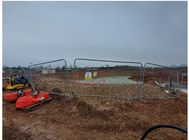
M7 towards northwest – Burrow pit in the northern part of the site has been securely fenced to mitigate risks associated with deep water and potential falls from height.
