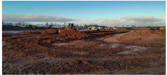
Grid W;6 towards North-northwest – Trimming of overfill ready for rerolling and/or chemical treatment.
