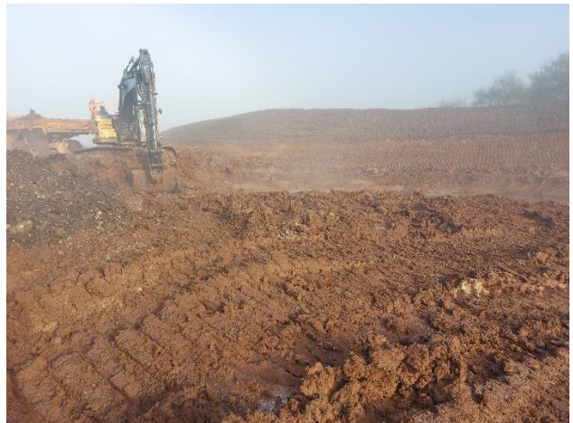
T12 towards north - Excavation at grids S11-S12 is ongoing.
