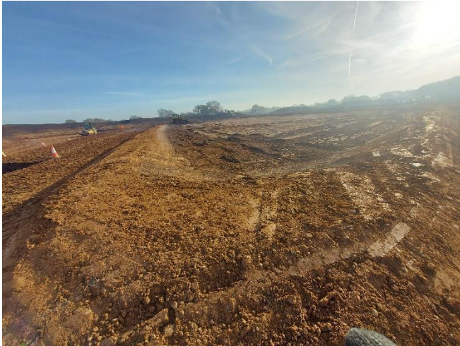
P6 towards south - An area being prepared at grids P7-P8 and Q7-Q8 to place the excavated material in bunds for screening.
