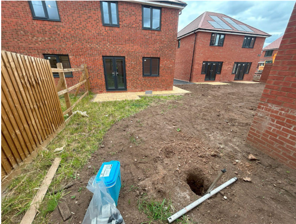
View of inspection pit in rear garden of Plot 195
