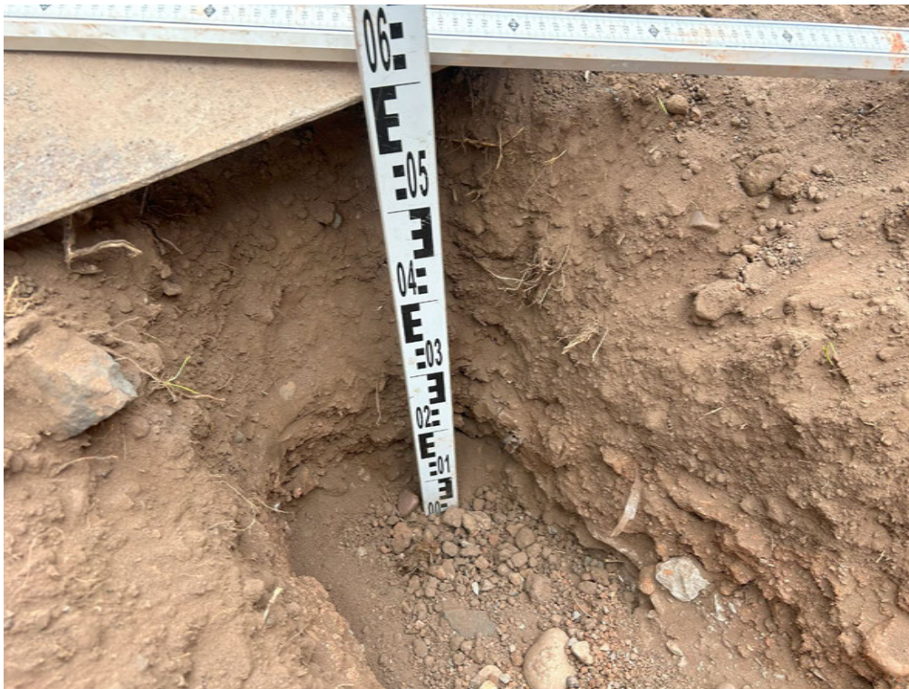
Depth of pit at Plot 167, proving a 600mm-thickness of clean cover system placed
