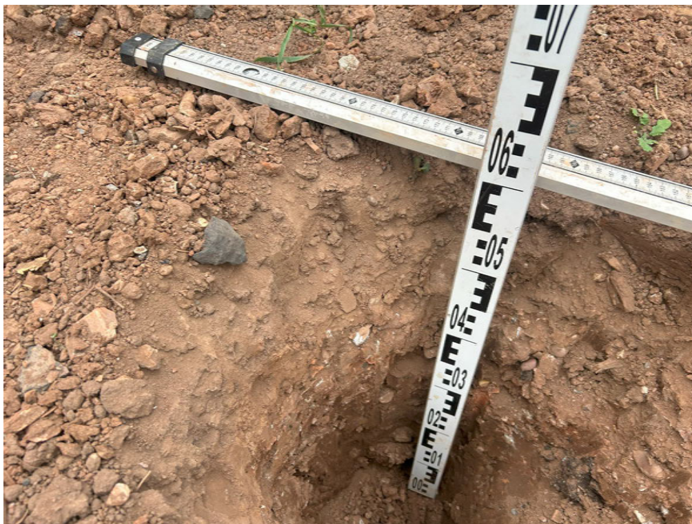
Depth of pit at Plot 184, proving a 600mm-thickness of clean cover system placed
