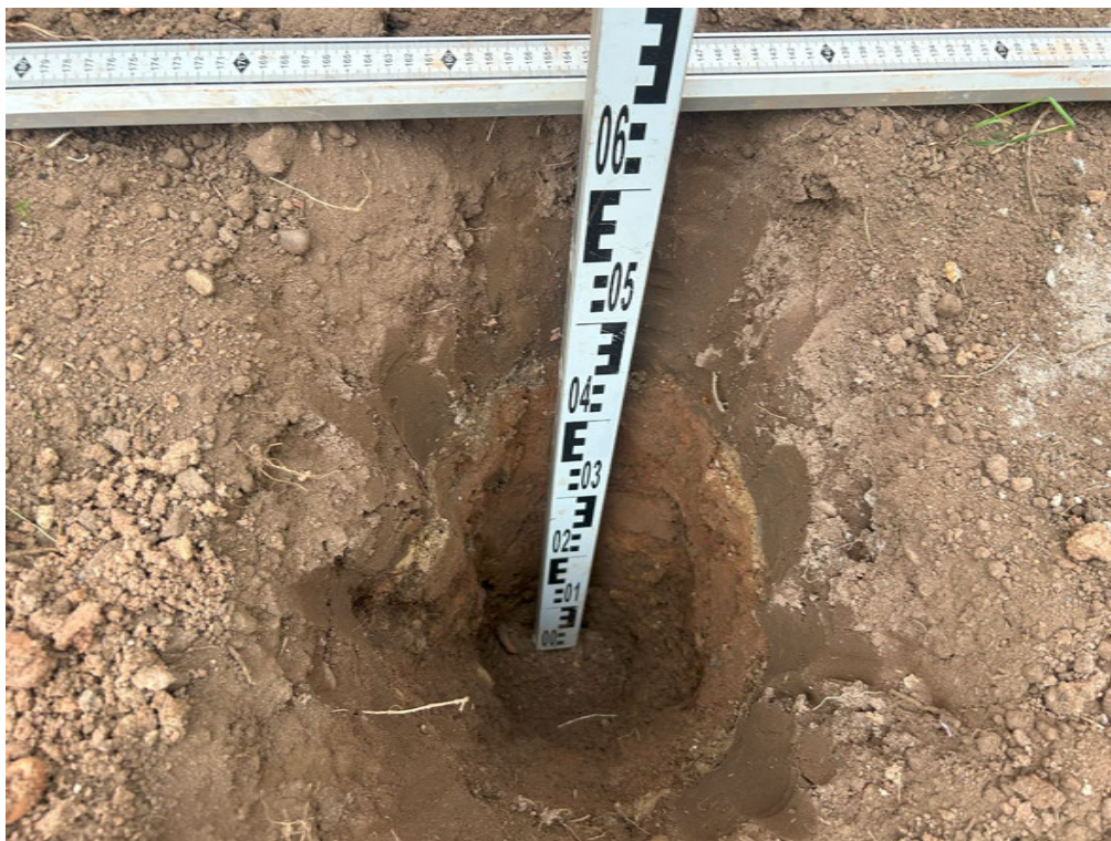
Depth of pit at Plot 195, proving a 600mm-thickness of clean cover system placed
