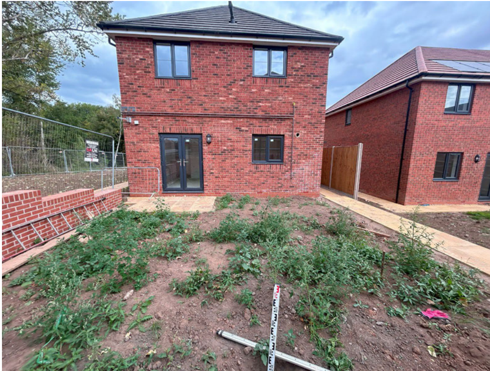
View of inspection pit in rear garden of Plot 200
