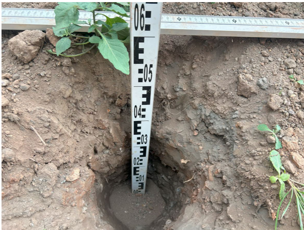
Depth of pit at Plot 200, proving a 600mm-thickness of clean cover system placed
