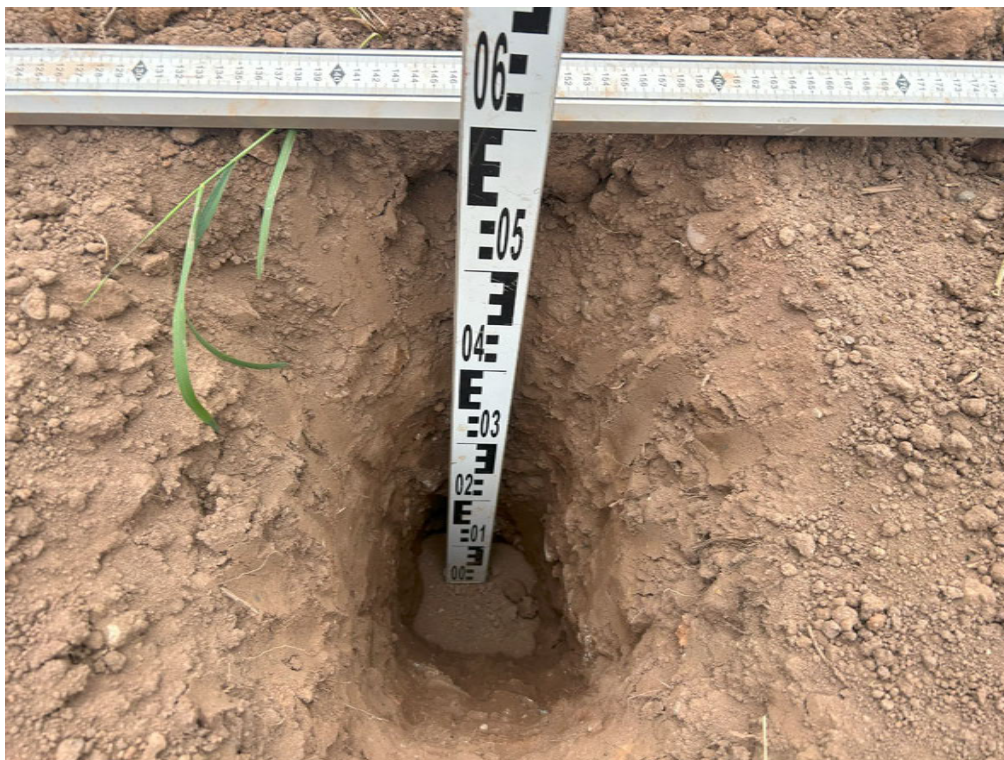
Depth of pit at Plot 192, proving a 600mm-thickness of clean cover system placed
