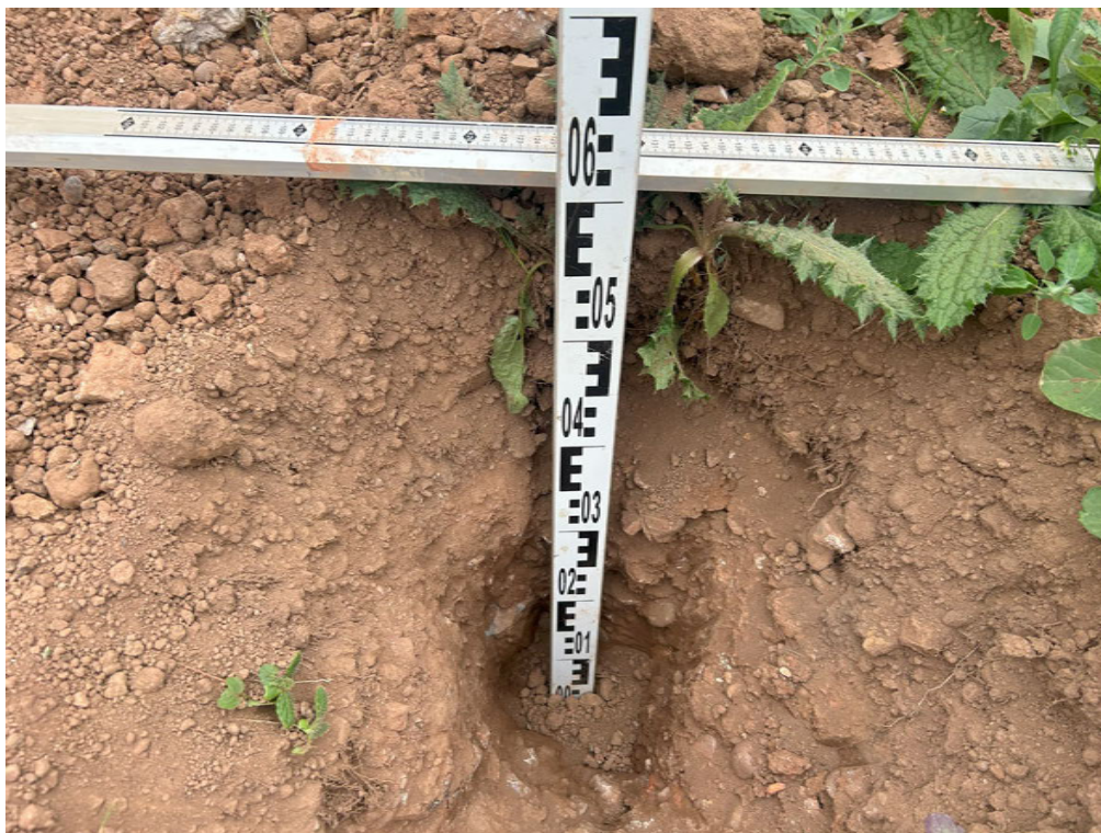
Depth of pit at Plot 180, proving a 600mm-thickness of clean cover system placed
