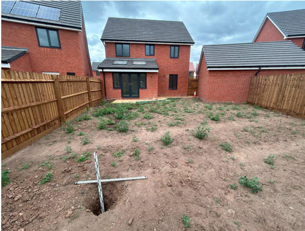
View of inspection pit in rear garden of Plot 184
