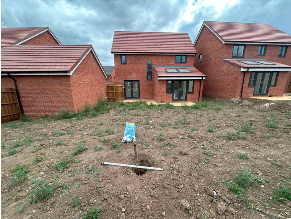
View of inspection pit in rear garden of Plot 188
