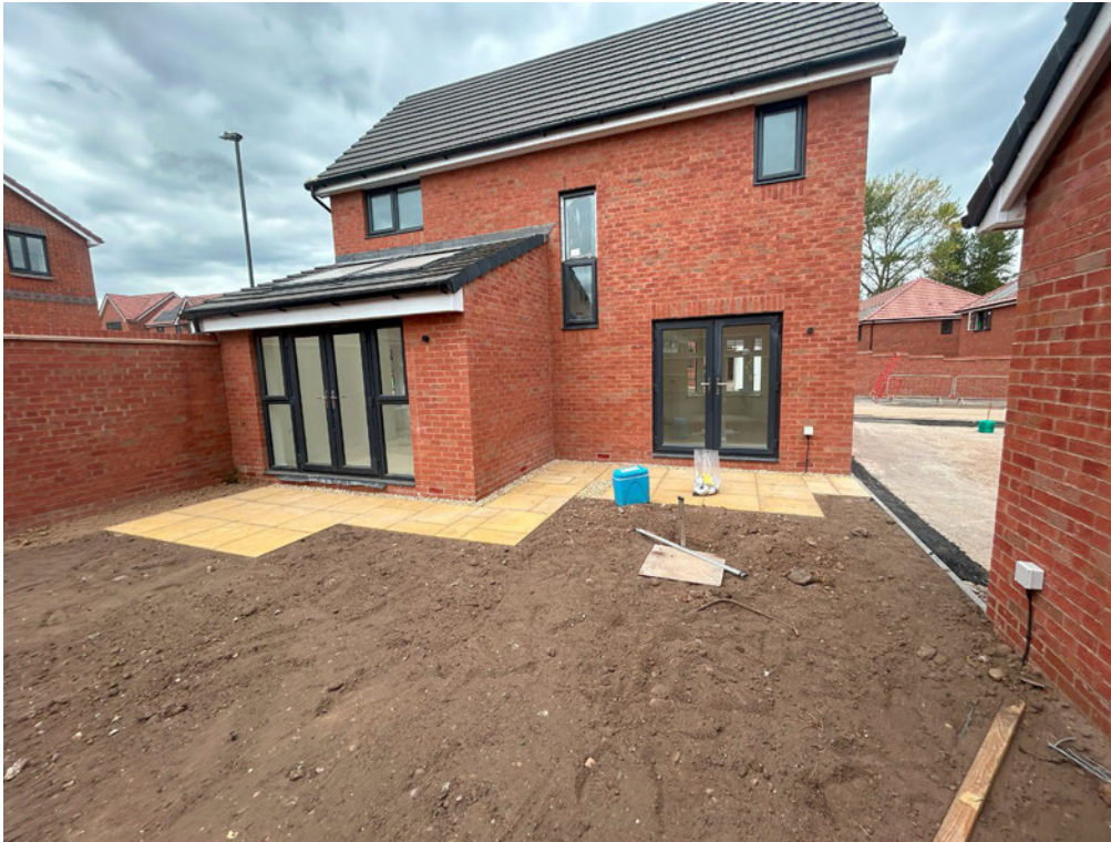
View of inspection pit in rear garden of Plot 167
