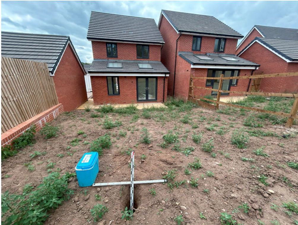
View of inspection pit in rear garden of Plot 192
