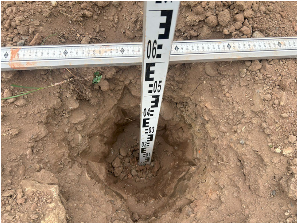
Depth of pit at Plot 188, proving a 600mm-thickness of clean cover system placed
