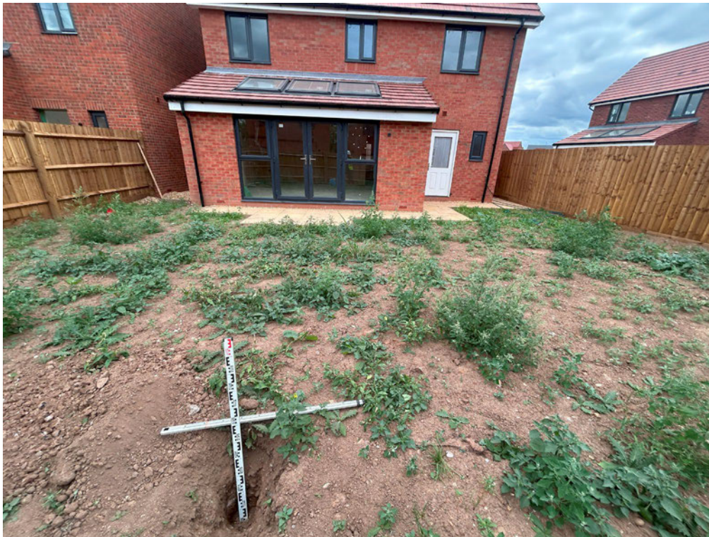
View of inspection pit in rear garden of Plot 180
