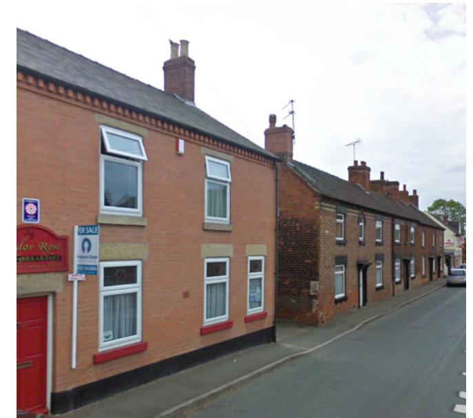
Red brick with stone lintels and cills. Some decoration at eaves level.
