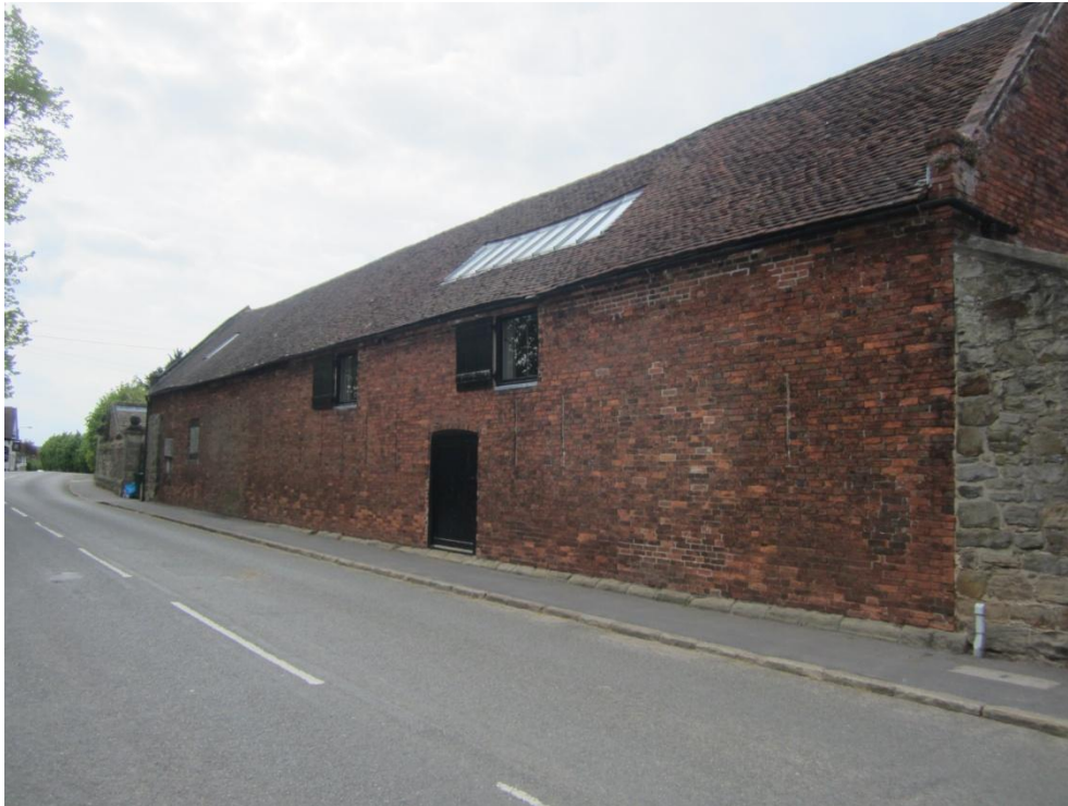
1. The outbuildings of Kings Newton Hall are a striking but plain feature of the street scene.
