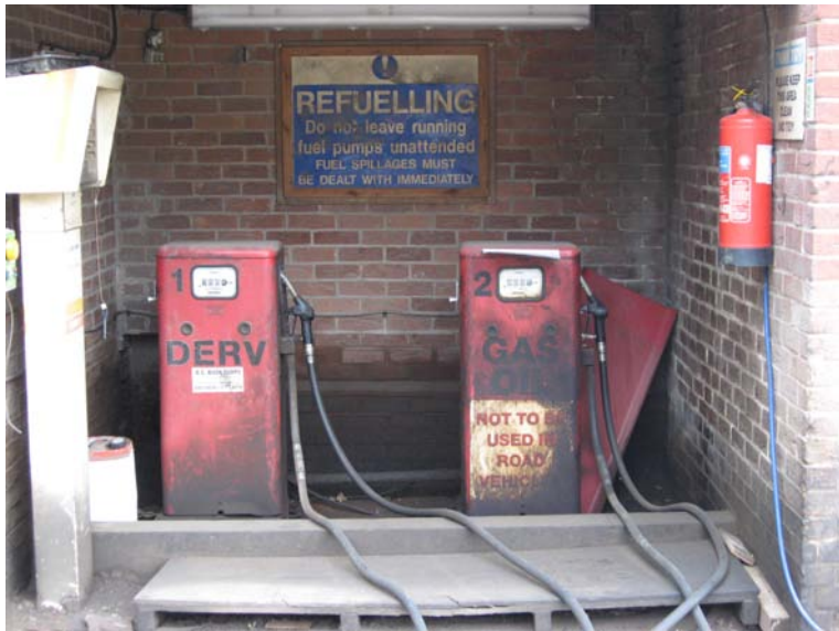
Plate 31: Old diesel dispensers in central area of site
