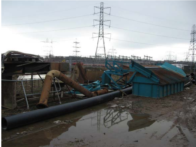
Plate 17: Plant storage to east of the site
