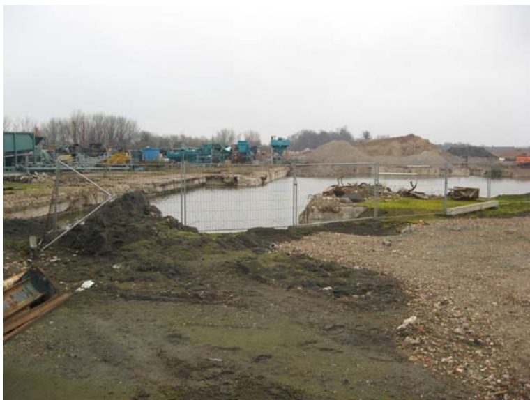
Plate 8: Aggregates processing pond, on site
