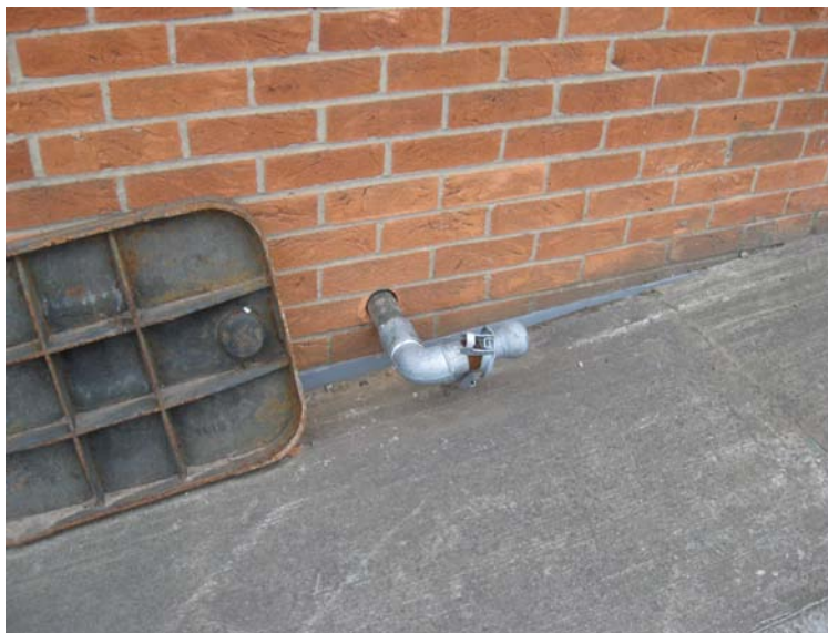
Plate 28: Unbundled pipework protruding from substation in central area of site
