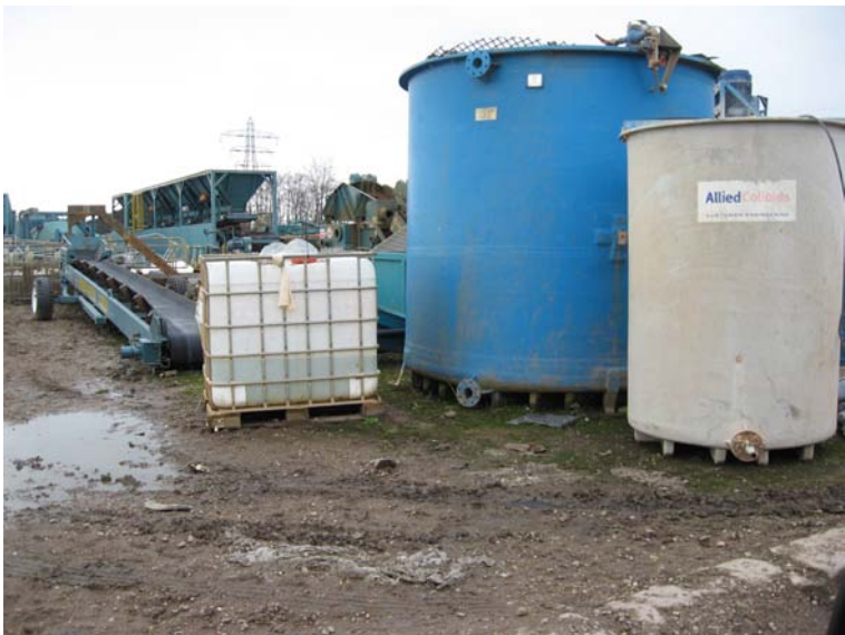
Plate 16: Hazardous chemical storage in west of the site
