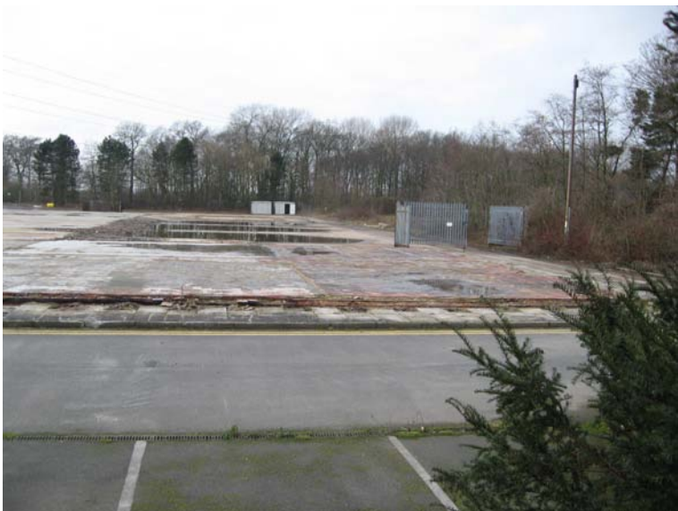
Plate 32: Demolished building footprint in south of site
