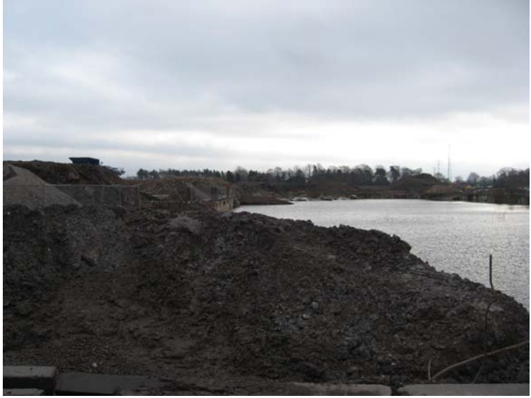
Plate 18: Stockpiled aggregates and process lake to west of the site
