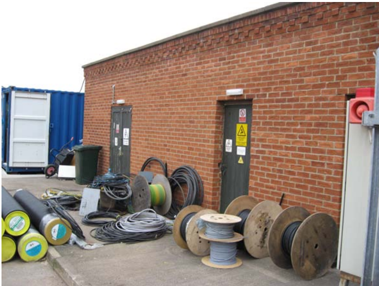
Plate 27: Electrical cable etc stored outside substation in central area of site
