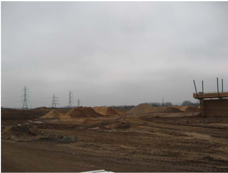
Plate 23: Stockpiling of materials and earthworks to south-central area of site
