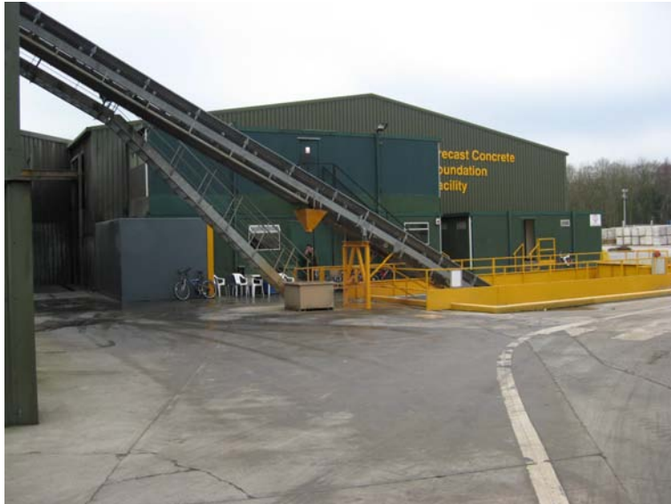
Plate 5: Foundation fabrication sheds, on site
