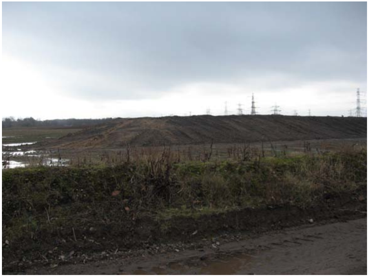
Plate 14: Stockpiles of material to centre of the site
