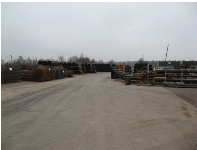
Plate 4: Storage of materials in the site
