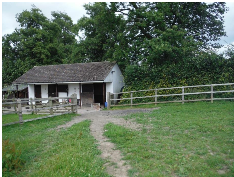
Photograph 2 –Disturbed ground at gate entrance
