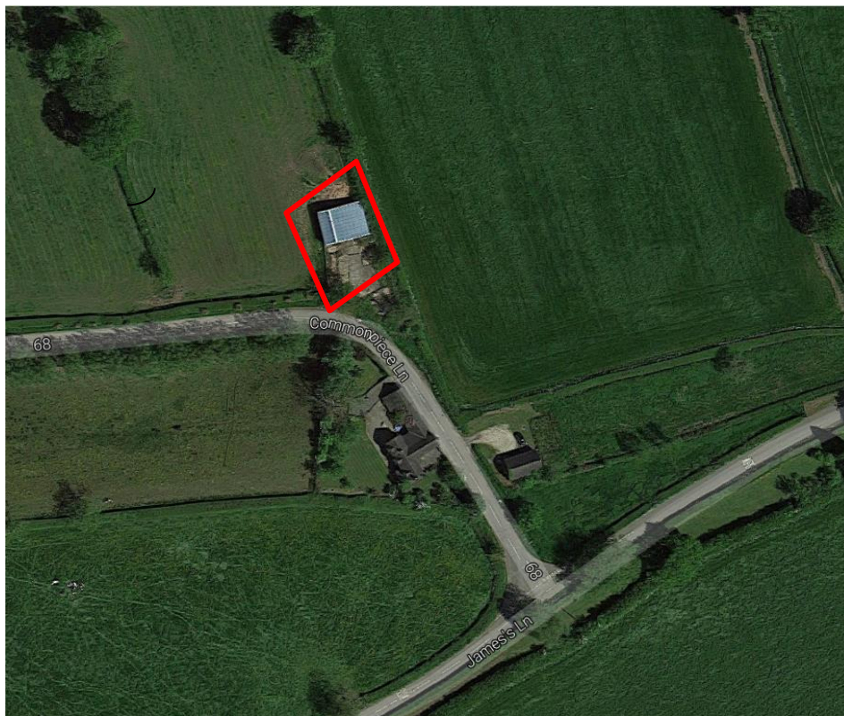
Aerial view – North ▲
