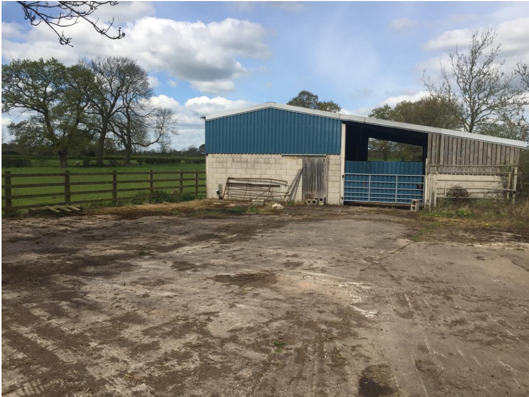
Approach from South - building facilitates livestock in fields to north-west, existing yard in foreground
