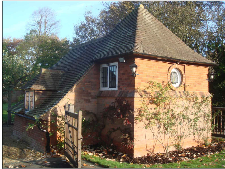
FIG 13. VIEW FROM THE FRONT EXTERIOR OF THE ENGINE SHED
