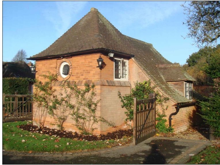
FIG 12. VIEW FROM THE FRONT EXTERIOR OF THE ENGINE SHED
