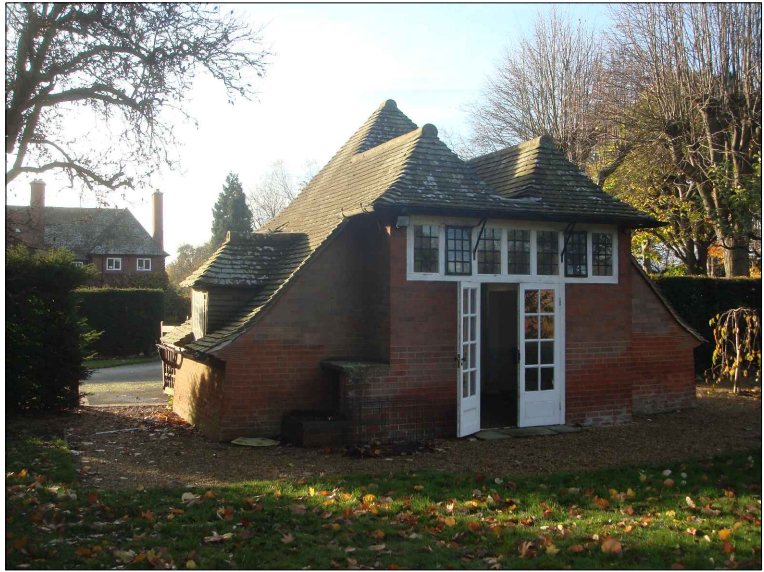
FIG 11. VIEW FROM THE REAR EXTERIOR OF THE ENGINE SHED
