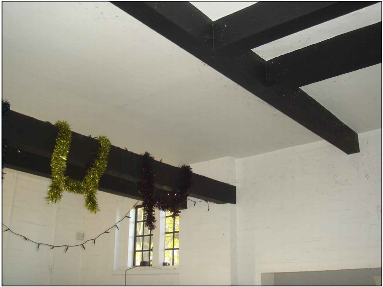
FIG 9. VIEW LOOKING UP AT THE EXISTING BEAMS
