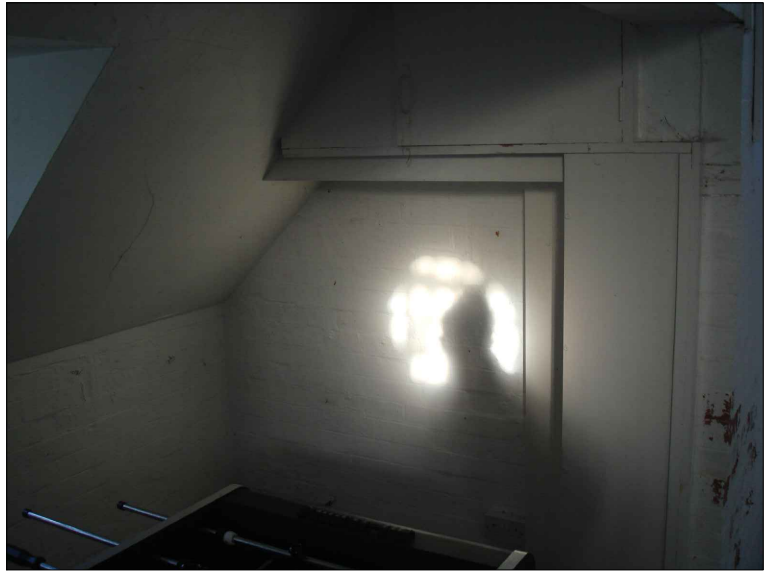
FIG 10. VIEW LOOKING INTO THE SPACE TO THE RIGHT HAND SIDE OF THE MAIN ROOM
