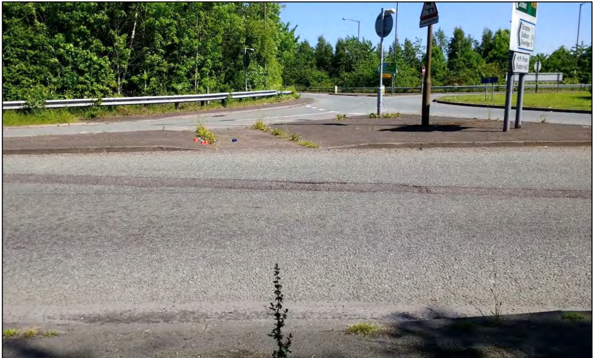
Figure 6 - Pedestrian Dropped Crossing
