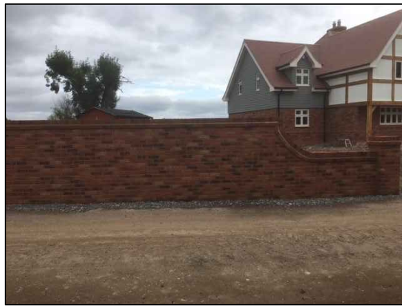
masonry brick wall is 13m long and 800mm high for 2.5m and increases to 1.5m for the remaining 10.5m.
