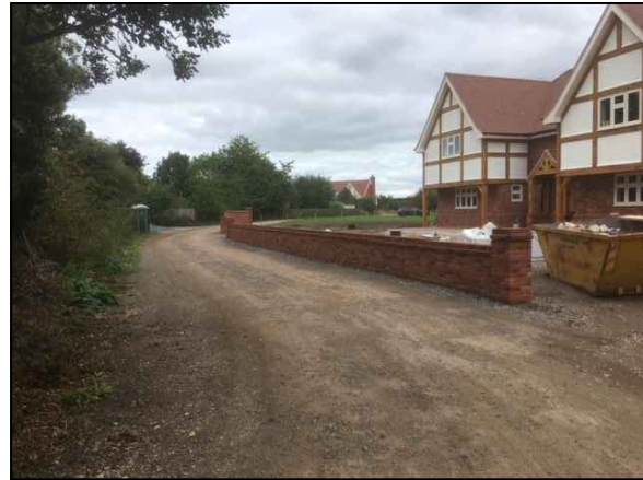
masonry brick wall is 24.6m long by 800mm high with 1.1m high pillars either side.
