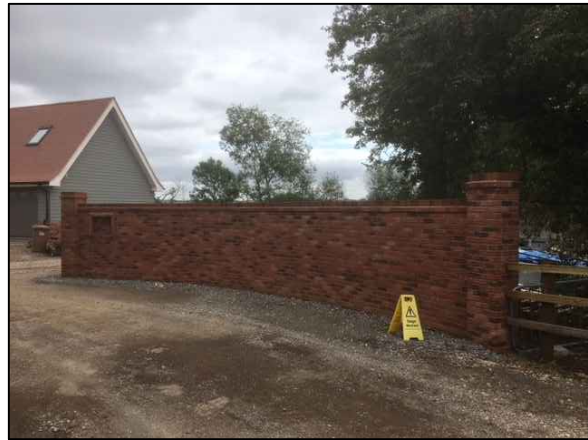
masonry brick wall is 11.5m long by 1.7m high.
