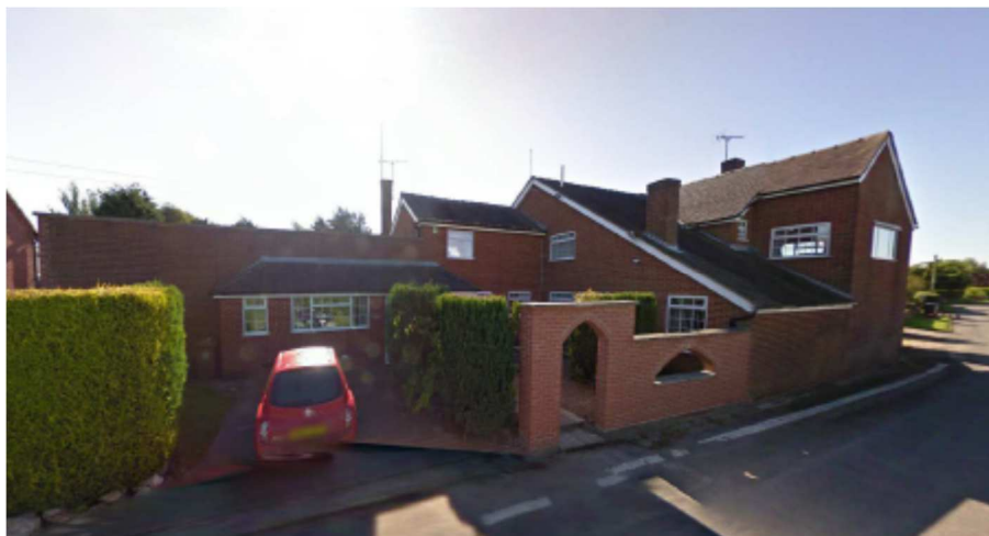
View to road showing parapet wall with hipped porch extension
