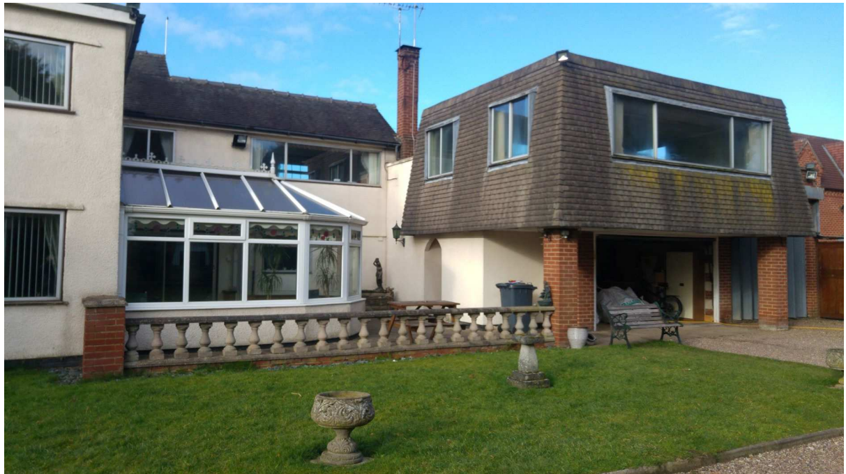
Back view with first floor extension over garage
