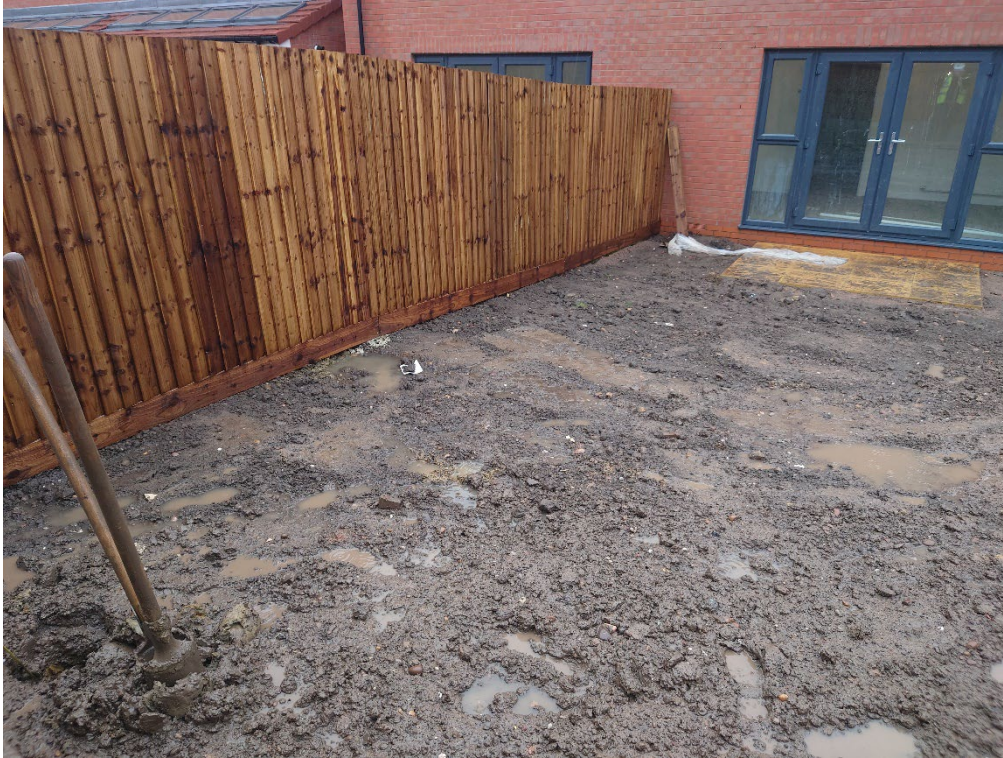
View of inspection pit in the rear garden of Plot 587
