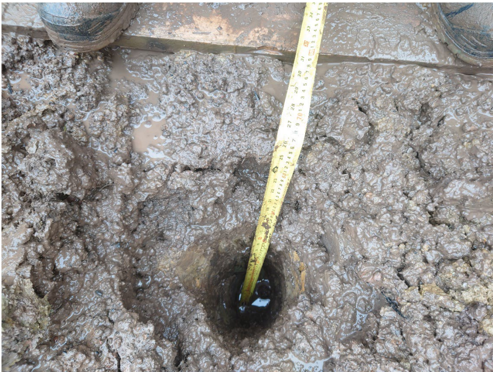
Depth of pit at Plot 581, proving 600mm-thickness of clean cover system placed
