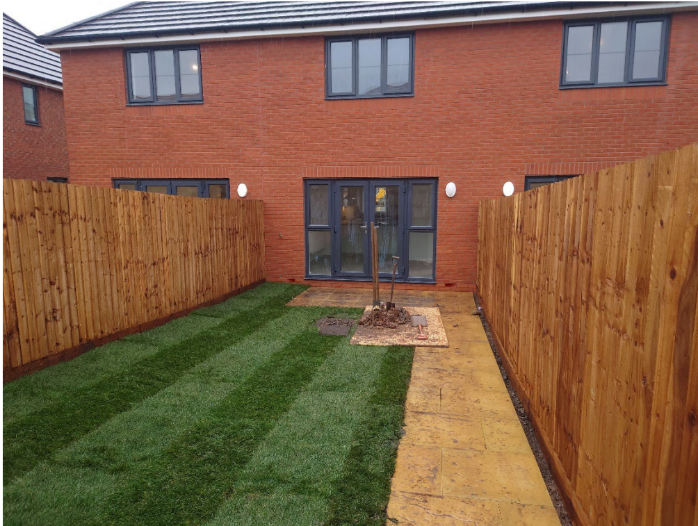
View of inspection pit in the rear garden on 582
