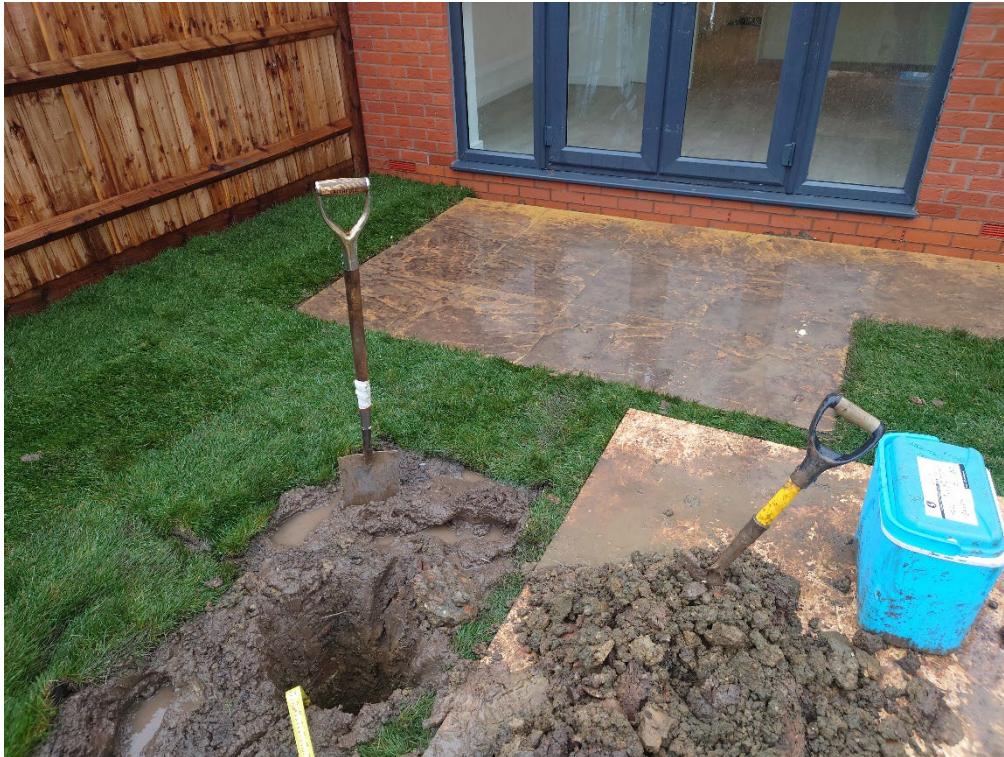
View of inspection pit in the rear garden of Plot 581
