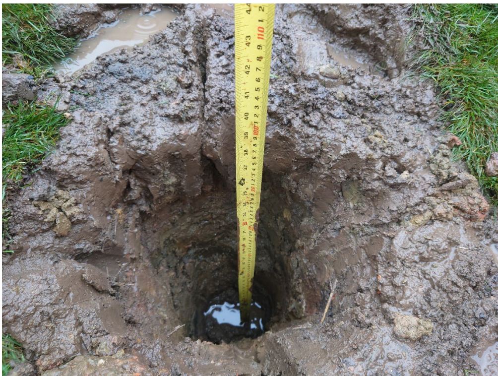
Depth of pit at Plot 581, proving 1000mm-thickness of clean cover system placed
