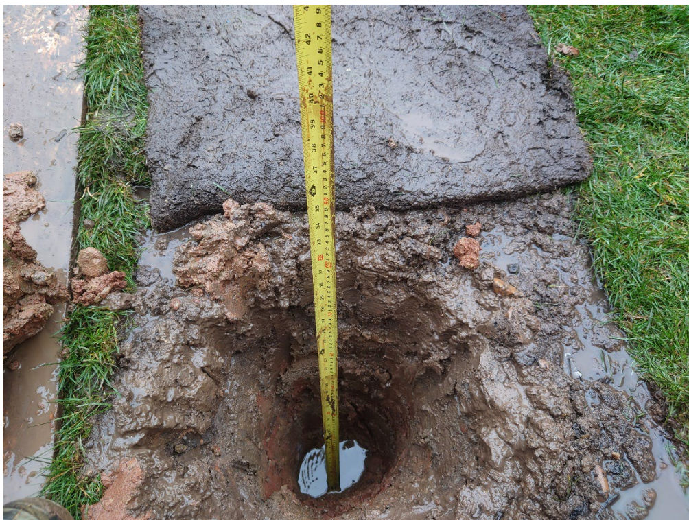
Depth of pit at Plot 582, proving 800mm-thickness of clean cover system placed
