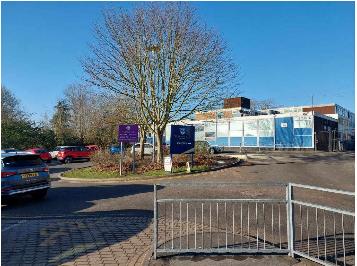
Location 40 - facing SW
