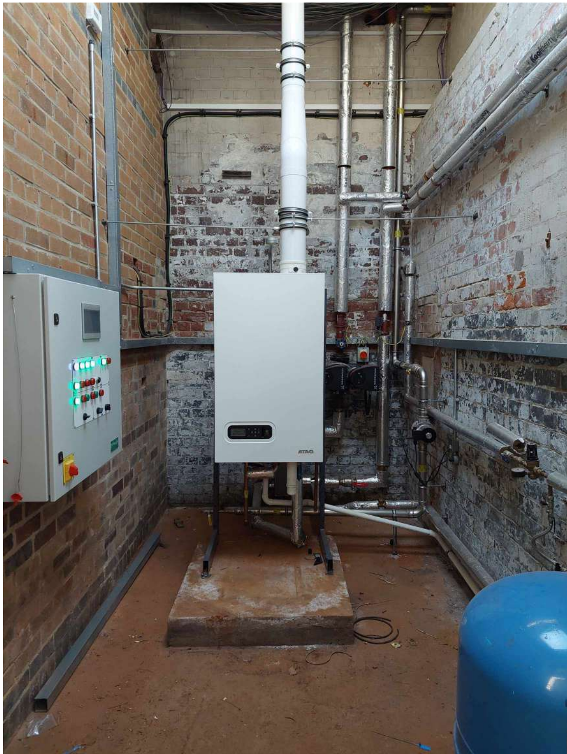
Location 45 - within boiler room
