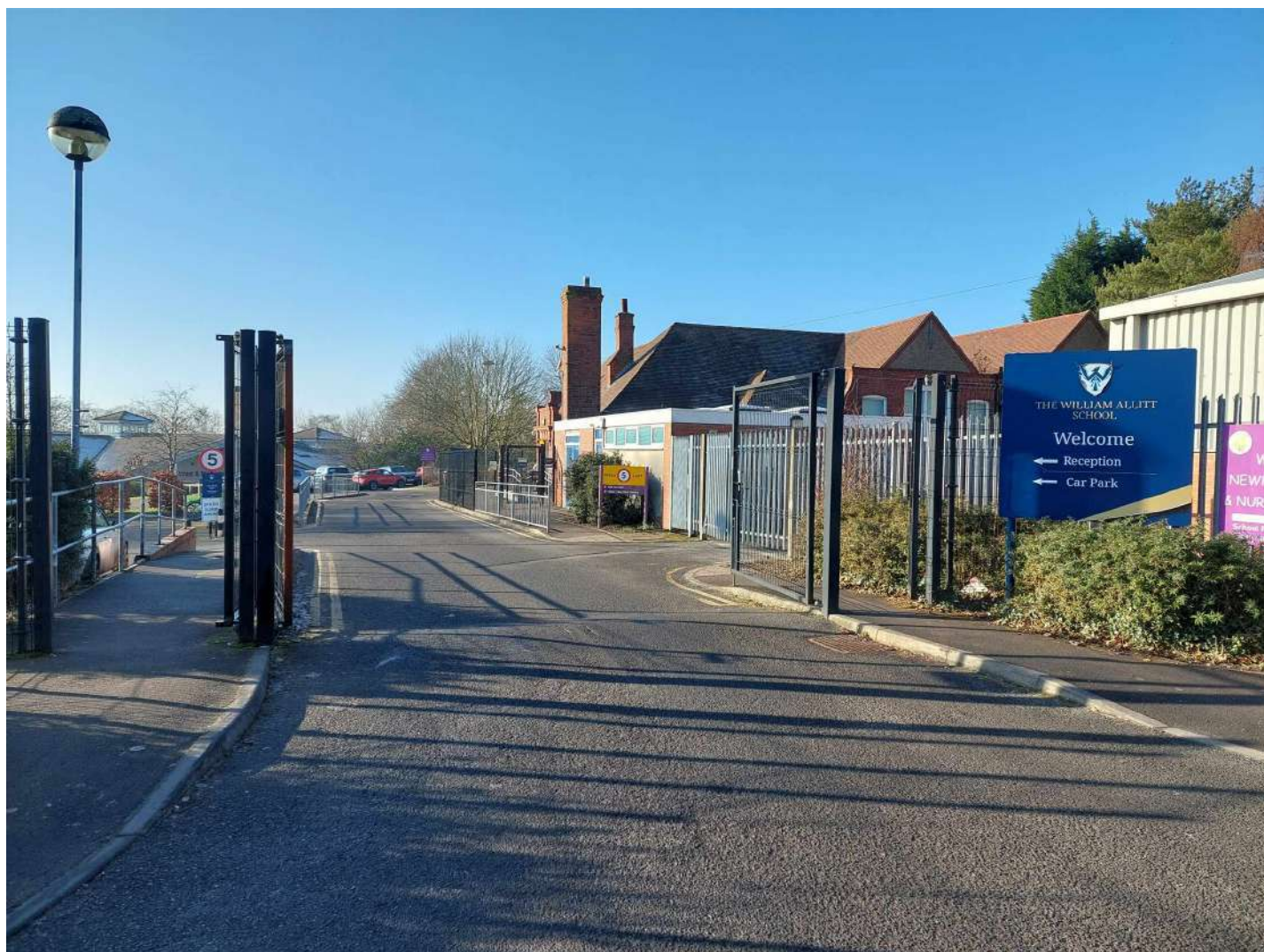
Location 43 - facing SW
