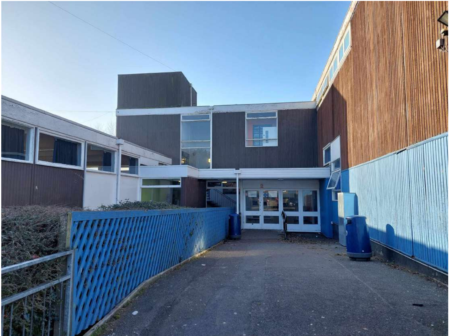
Location 38 - facing SW
