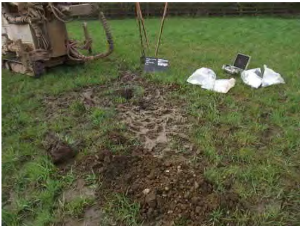
Borehole WS10: Prior to Rigging up on Completion of Starter Pit, Note the Marshy Ground.
