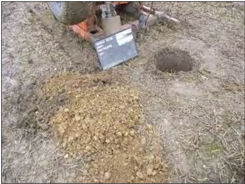
Borehole BH8: Starter Pit Spoil Heap.
