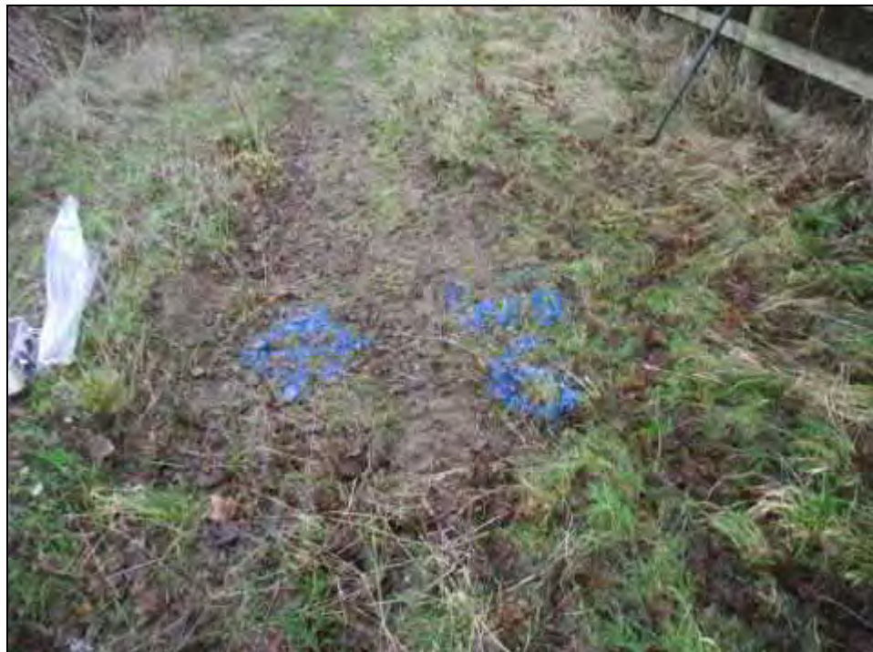
Borehole WS6: Prior to Rigging up.
