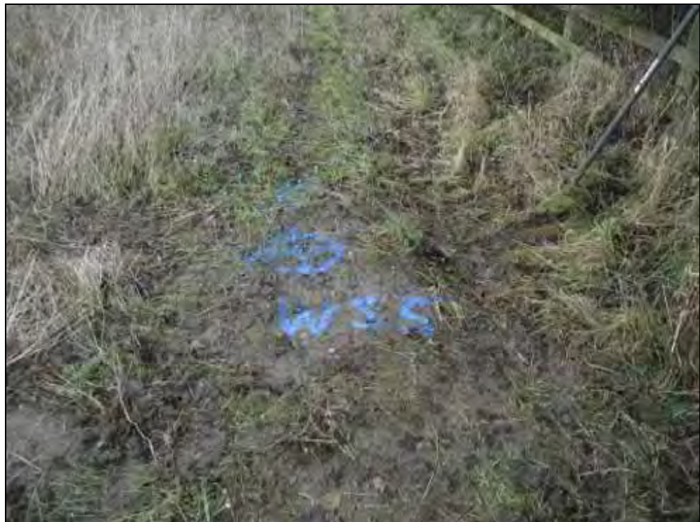
Borehole WS5: Prior to Rigging up.
