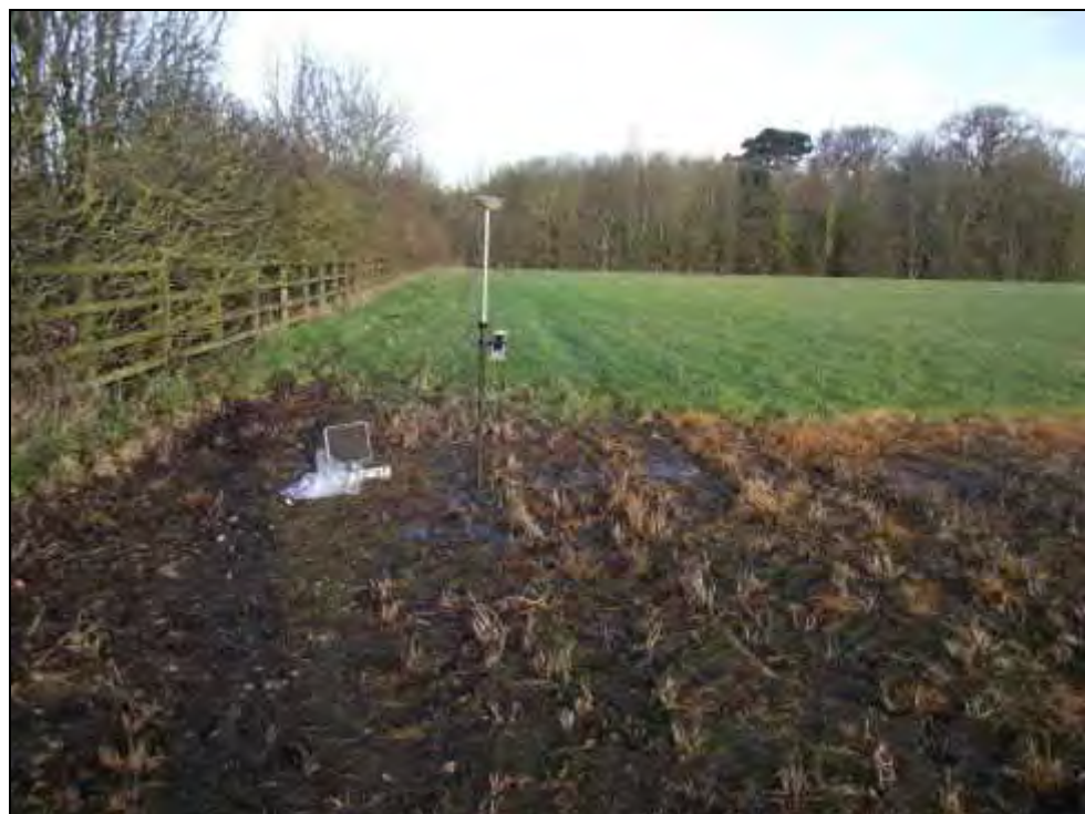
Borehole WS9: Prior to Rigging up Looking North.
