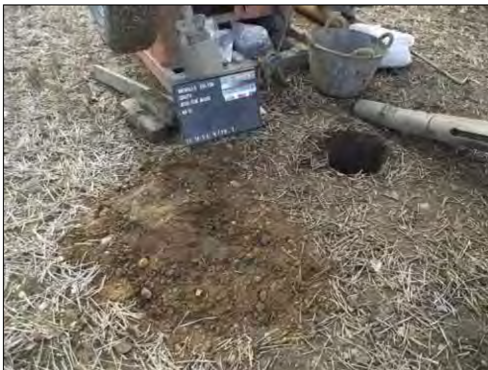
Borehole BH10: Starter Pit Spoil Heap.
