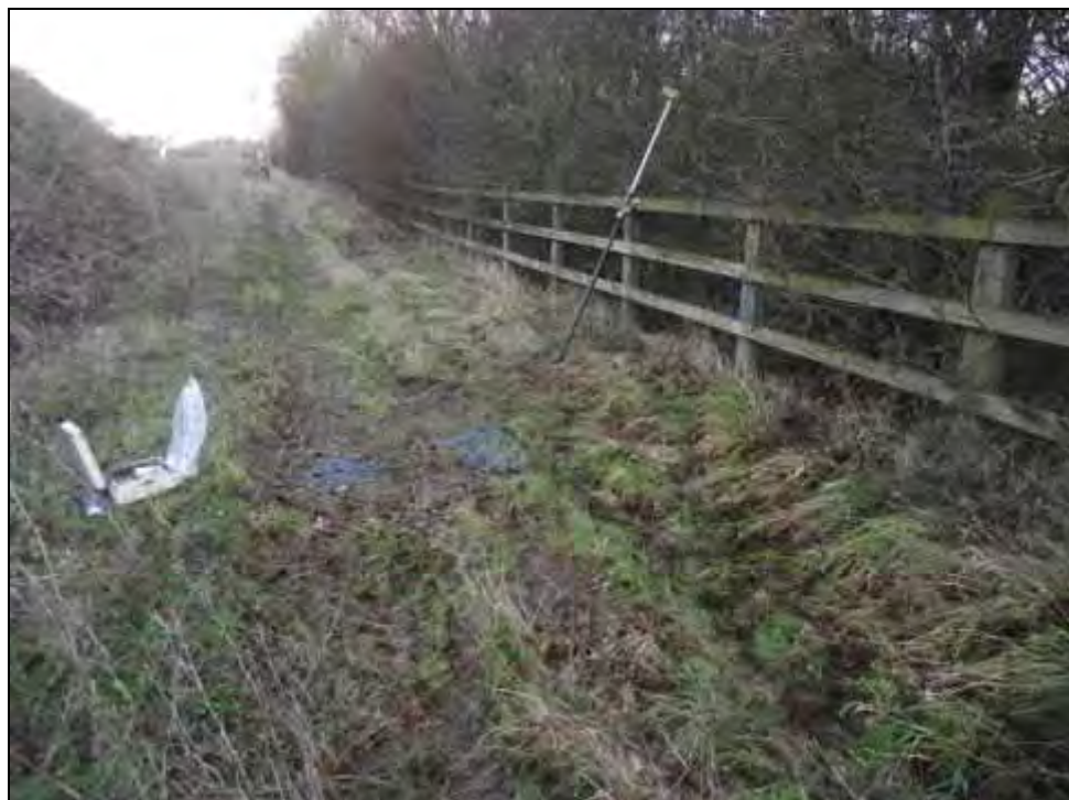
Borehole WS6: Prior to Rigging up Looking North.
