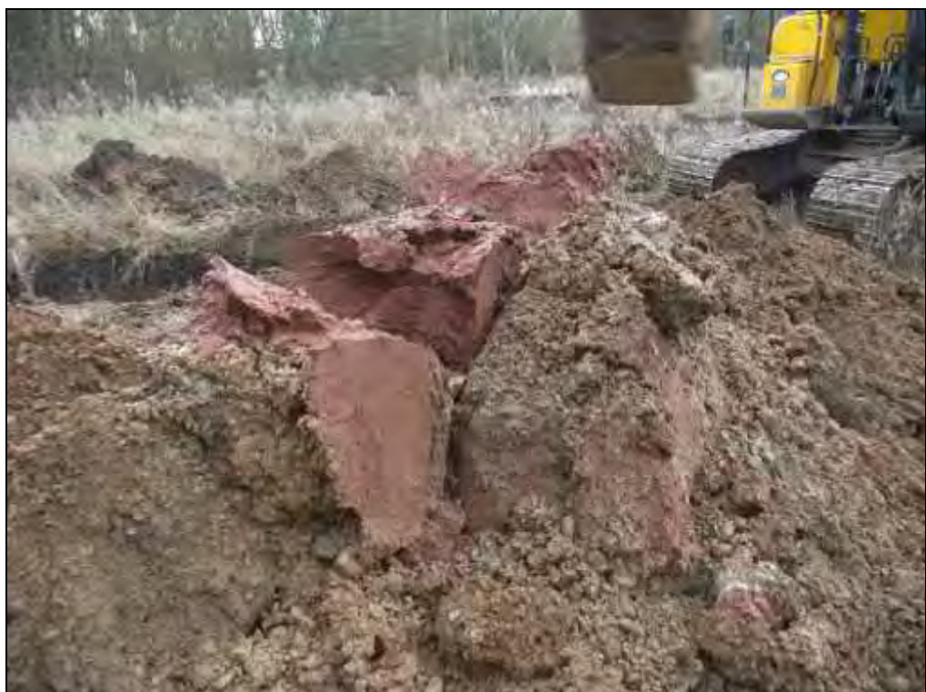
Trial Pit TT2: Spoil From North Western Section of Trench.
