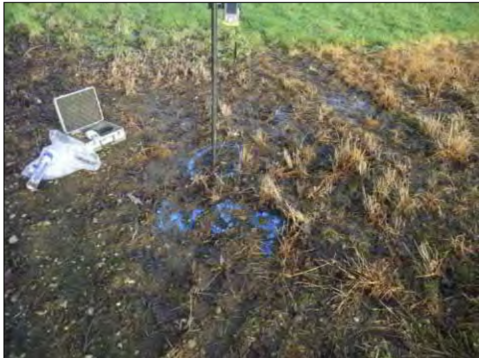
Borehole WS9: Prior to Rigging up.
