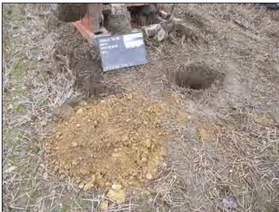
Borehole BH9: Starter Pit Spoil Heap.
