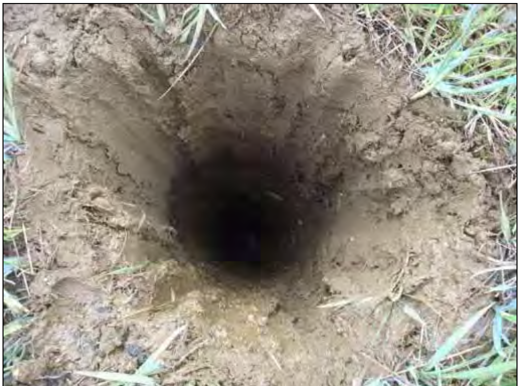
Borehole WS10: Close up of Starter Pit Plan View.
