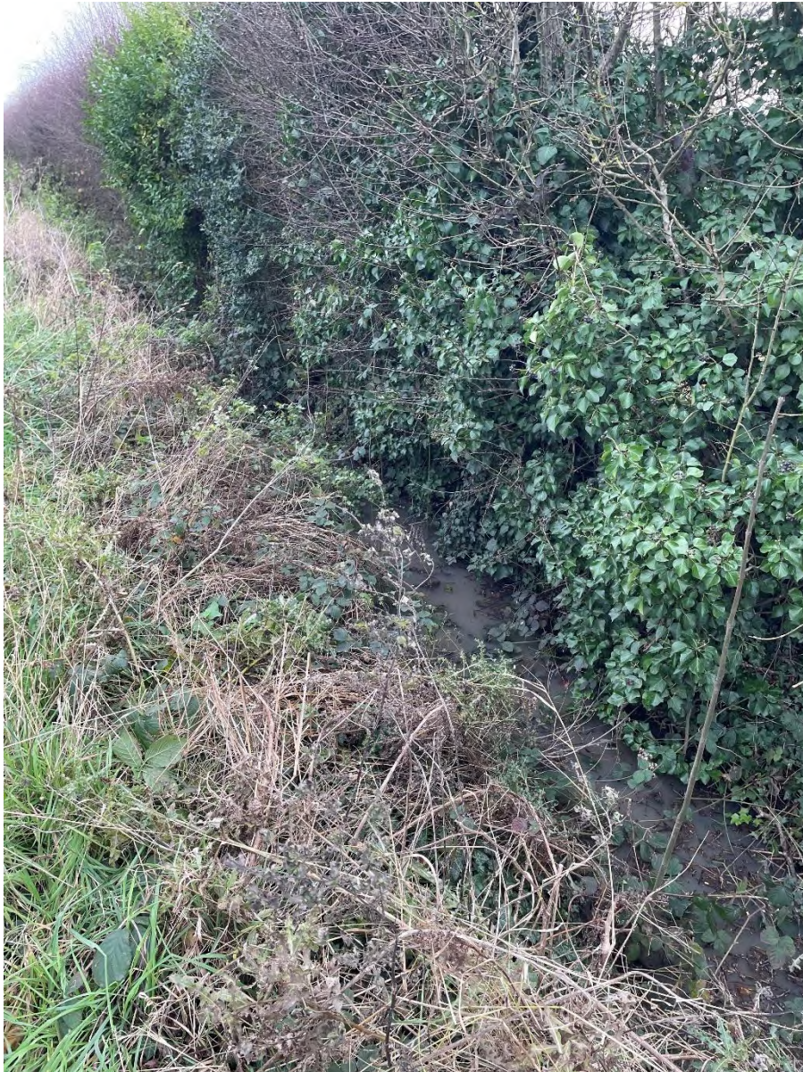
Figure 1.3: Drainage Ditch along Northern Boundary (December 2024)
